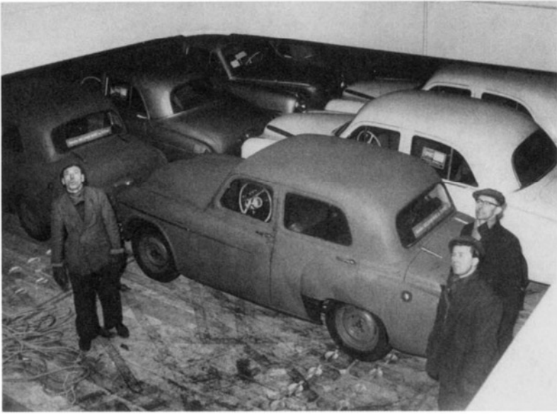
A general cargo vessel converted to carry cars, 1955 (photograph WWL Archive)
