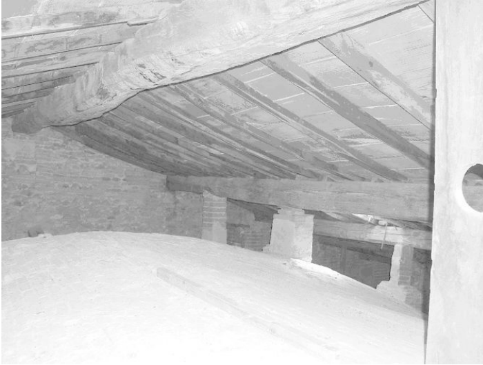
Figure 6. Extrados of the cross vault.
