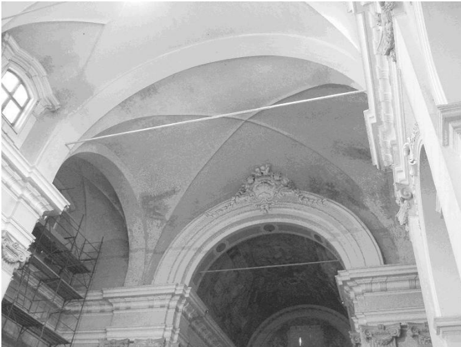
Figure 5. The roof vault of the presbytery area.
