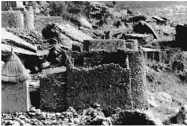
Figure 10.7 An abandoned compound, 1983
