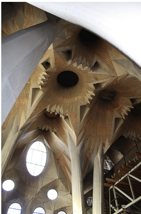
Figure 3.5 Sagrada Família. The domes and arches at the Sagrada Família are all based on hyperbolic paraboloids which results in a very lightweight structure compared to the early Romanesque semi-circular forms. © Dennis Sharp
