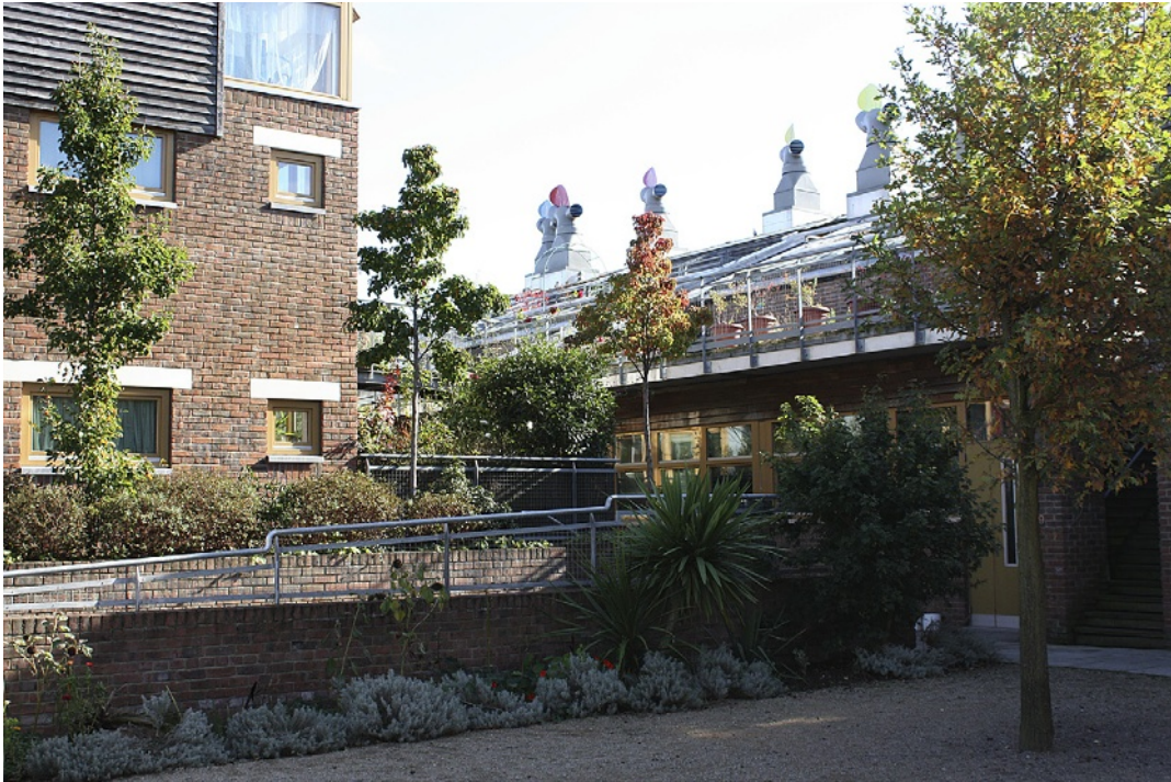
Figure 1.8 Bedzed (2002). The innovative award-winning eco-housing scheme by Bill Dunster Architects in Beddington, South London. Wind cowls on the roof ventilate the houses; photovoltaics power electric cars; sun spaces and a high thermal mass are part of the low-energy strategy of this design. © Dennis Sharp
