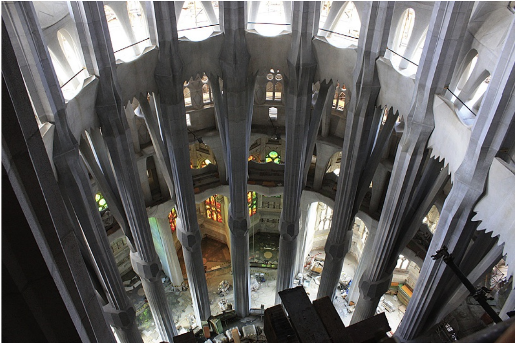
Figure 1.6 Sagrada Família (1882). Gaudi's major work, the Sagrada Família, is only just being completed, some 80 years after his death. The hyperbolic paraboloid geometry used in the structure is unique and inspirational. It is at the heart of Barcelona's enormous tourist industry that has evolved from Antonio Gaudi's architecture. It is a building designed with love and genius that brings enormous joy and love. © BookArt
