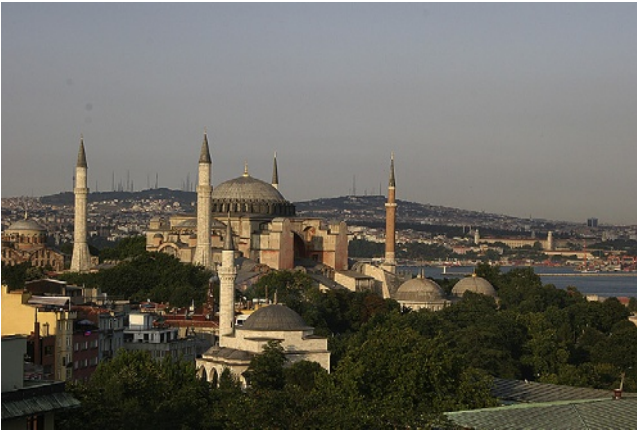
Figure 3.4 Hagia Sophia. This is one of the largest early domed structures. The original dome collapsed in 557AD after an earthquake and it was rebuilt with 40 braces and made slightly taller. The length of clear span of the 32 m central dome and the semi-domes was unprecedented at the time of Hagia Sophia's construction. To the northeast and southwest, in contrast, heavy double arches and pier buttresses were erected to counter the thrust of the dome.
