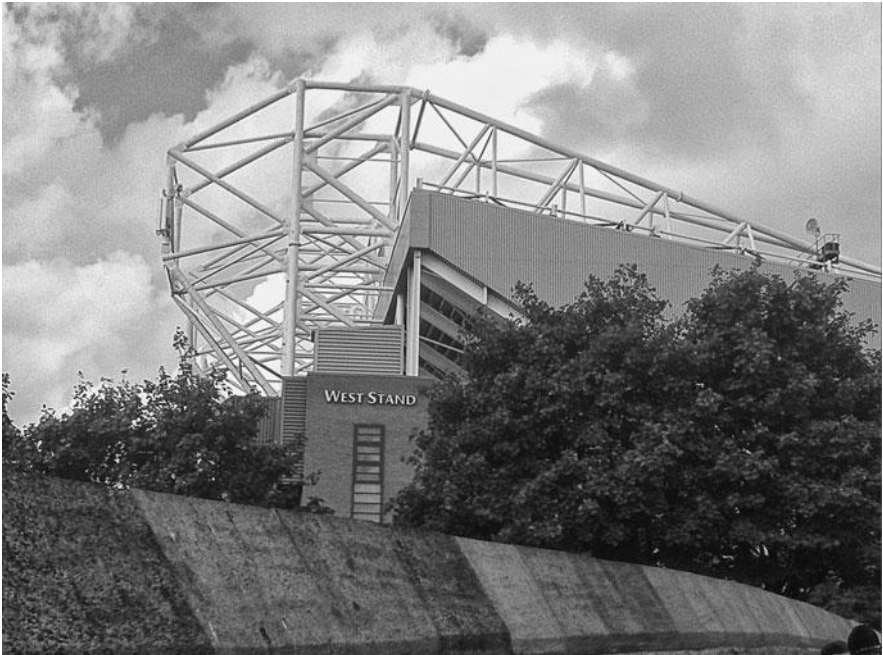
Figure 8.4 Old Trafford Stadium, home to Manchester United Football Club, and the cantilever roof structure, which is made from steel ( www.manutd.com )
