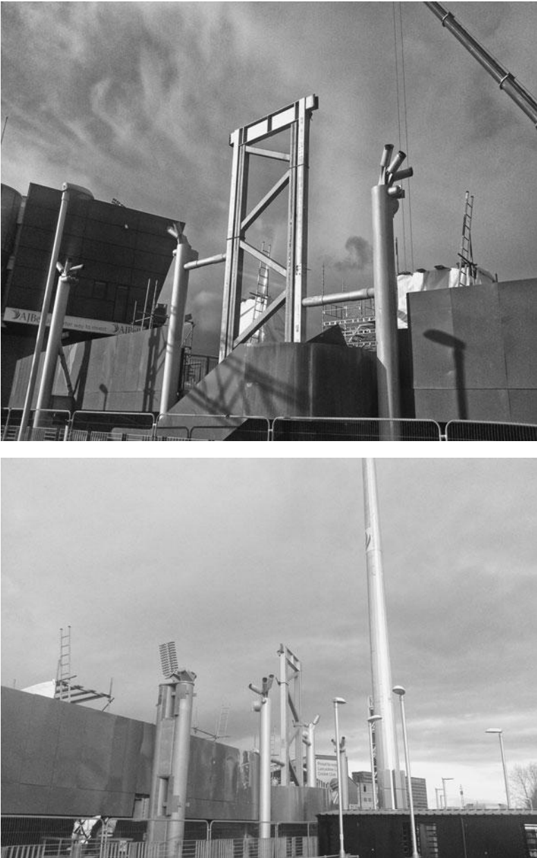
Figure 8.9 Prefabricated steel structures at the Emirates Old Trafford Cricket Ground, Manchester
