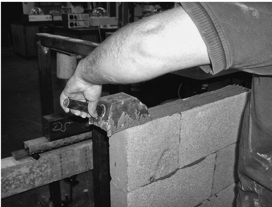
Figure 13.4 Application of thin layer mortar
