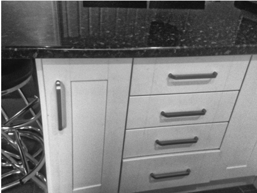
Figure 15.5 Melamine kitchen worktop
