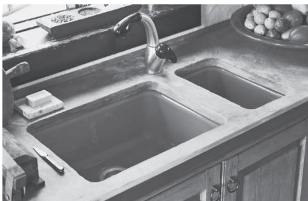
Figure 4-10b Two single-basin cast iron sinks used in combination (an undercounter installation in this example).
