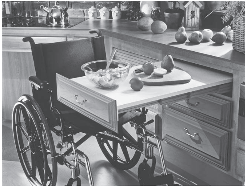
Figure 4-29b This pullout table provides a work surface for seated use.
