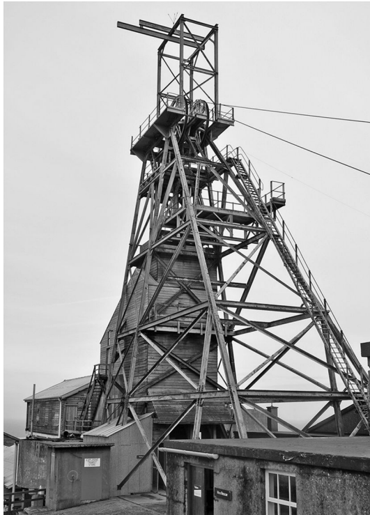
FIGURE 3.1 The headframe above the Victory shaft at Geevor Mine in Cornwall, England. Courtesy of Nilfanion under Creative Commons License.
