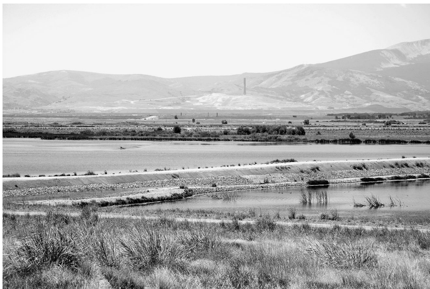
FIGURE 11.2 View of the Warm Springs Ponds to the southwest showing Pond 2 ( right ), Pond 3 ( left ), and the earthen embankment between them that impounds Pond 3. The Mill-Willow Bypass flows from left to right along the far side of the Warm Springs Ponds. Note the stack of the Washoe smelter at Anaconda in the distance near the center of the photo. Photo by the author.
