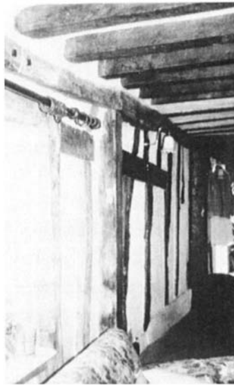
Plate 3b A medieval hall with inserted post and ceiling at Oaklands, Stanstead.
