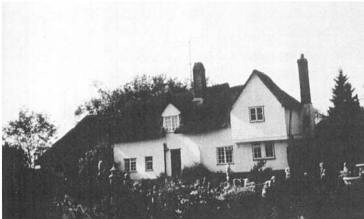
Plate 3c Highbank, Brent Eleigh: an open house with jettied wing.
