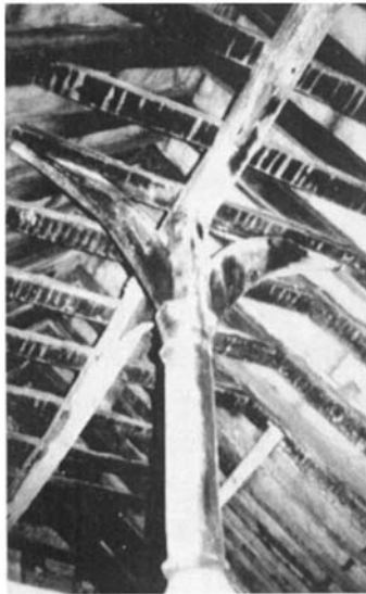
Plate 3a A crown-post roof with sooted timbers at Layers Breck, Rougham.
