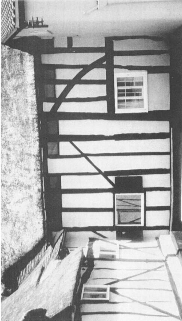
Plate 5c 42 Egremont St, Glemsford: contrast between 16th-century and later framing.
