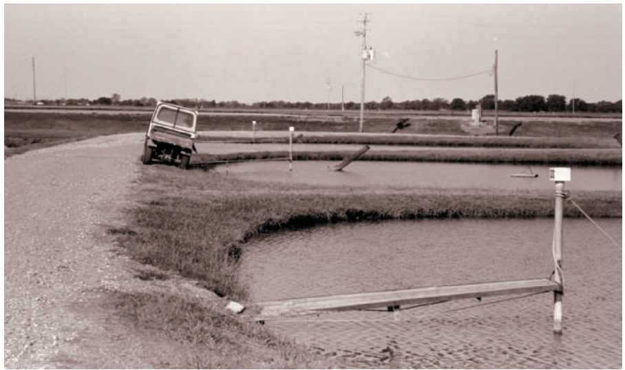
FIGURE 13-10 The modified Canfield outlet or inside swivel drain controls the water level by pivoting the drainpipe up or down on its swivel joint.
