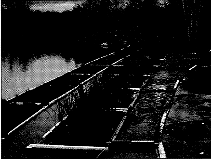
Figure 5.3 Floating cattails in mine drainage water provide nutrients for reducing bacteria that live in the root zone and sediments of the water.
