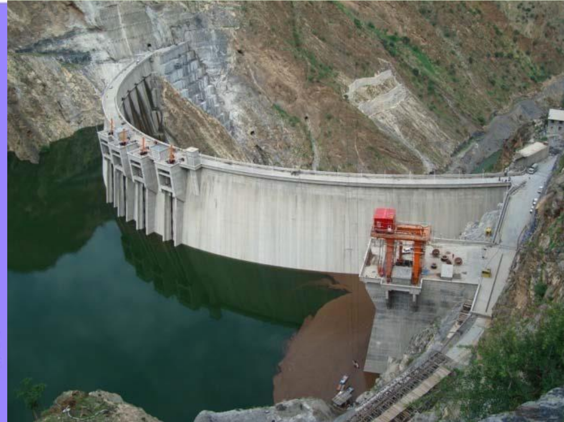
Arch Dam upstream view
