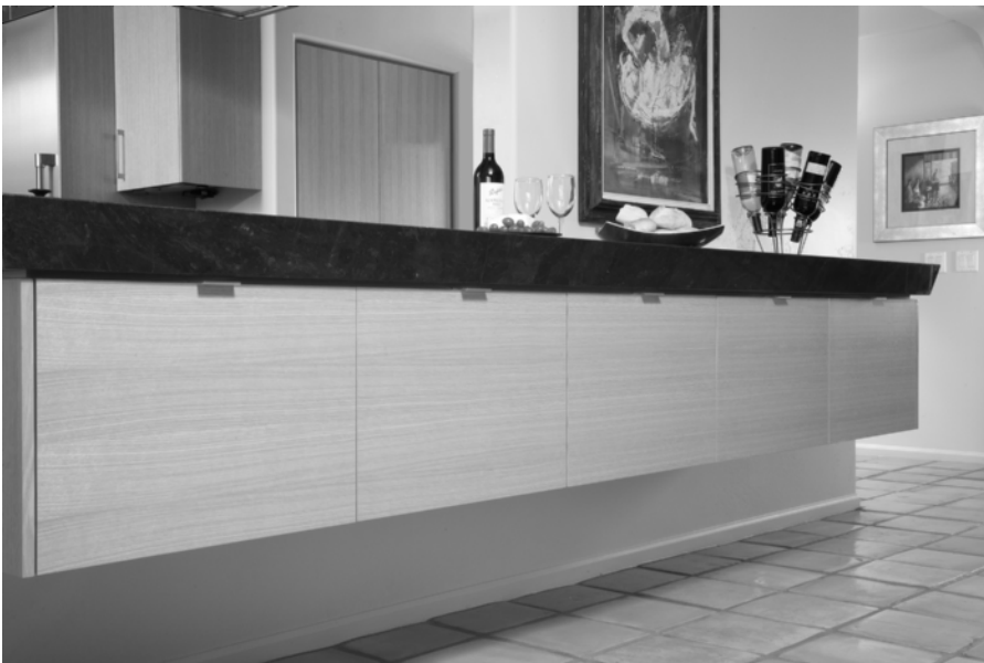
Figure 6-3 The advantage of the frameless construction style is access to cabinet interior space. (Photo courtesy of Mary Fisher Designs.com, Northlight Architectural Photography.com)
