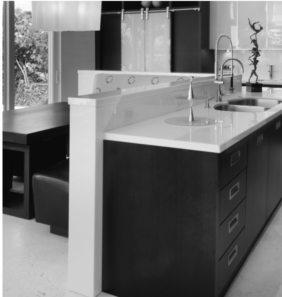
Figure 2-6 The pony wall is used to secure island cabinets and provide structure to run plumbing and electrical in the island. (Photo courtesy of Downsview Kitchens, www.downsviewkitchens.com )
