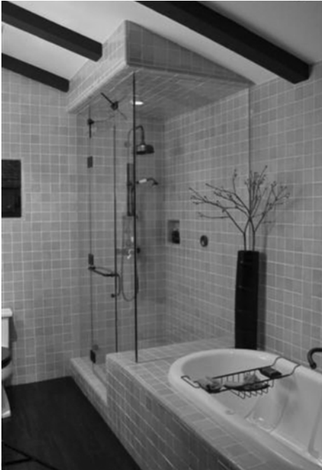
Figure 7-26 Steam showers must be fully enclosed to be properly functional. (Photo courtesy of David Dalton, Inc., Los Angeles, www.daviddaltoninc.com )
