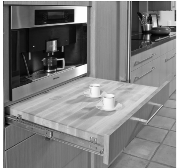
Figure 4-65 To provide landing space for the center, a pull-out board that locks into place was installed below the coffee center. (Photo courtesy of Mary Fisher Designs.com, Northlight Architectural Photography.com)
