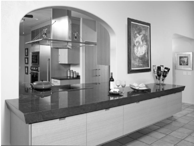
Figure 4-66 Cabinetry for the dry bar was anchored to the wall at every stud to carry the weight of the cantilevered cabinetry and granite countertop. The 3-inch, reversed-bevel counter edge detail adds additional impact to the look of the space. (Photo courtesy of Mary Fisher Designs.com, Northlight Architectural Photography.com)
