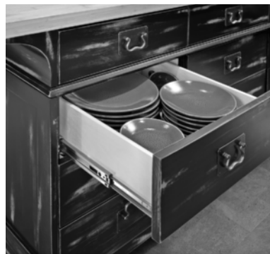
Figure 4-54 Drawers fully extend in the island to house dinnerware. (Courtesy of Judy Svendsen, ASID, Raven Interiors/Mary Fisher Designs.com)
