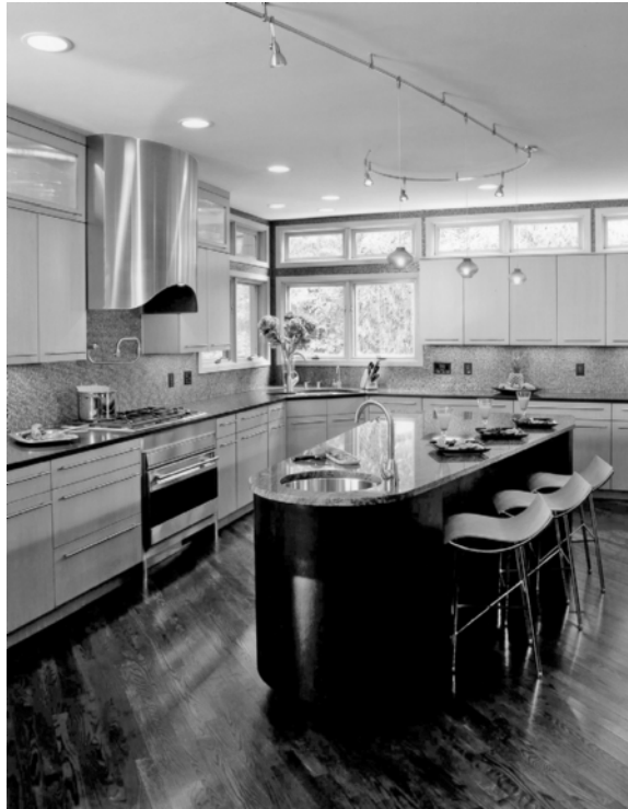
Figure 4-21 When a remodel has insufficient space to install a remodel recessed can, a track lighting system may be the solution. (Photo courtesy of Sub-Zero/Wolf Photograph)
