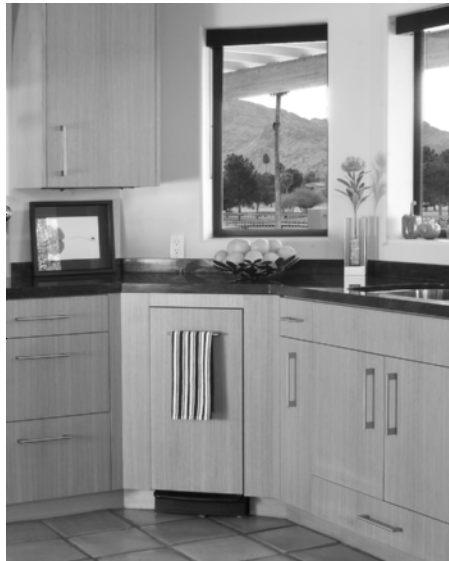
Figure 5-41 Trash compactors can be specified to receive cabinet panels or finished fronts. (Photo courtesy of Mary Fisher Designs.com, Northlight Architectural Photography.com)
