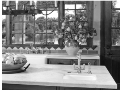
Figure 4-26 Undermount sink. (Photo courtesy of Northlight Architectural Photography.com, Mary Fisher Designs.com)
