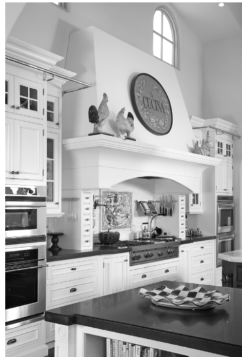
Figure 5-34 The most important aspect in the selection of a ventilation system is the capture area. (Photo courtesy of Mary Fisher Designs.com, Northlight Architectural Photography.com)
