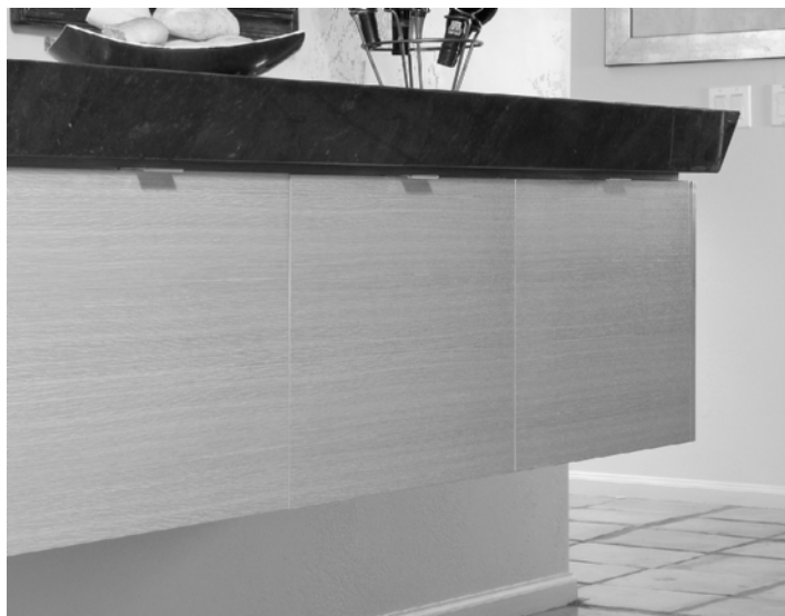
Figure 4-36 Some edge details, such as a reverse bevel edge, may extend more than 1-1/2". (Photo courtesy of Mary Fisher Designs.com, Northlight Architectural Photography.com)
