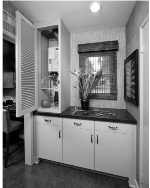
Figure 4-56 New cabinet storage and counter surface were created in space previously lost to the water heater tank. (Courtesy of Judy Svendsen, ASID, Raven Interiors/Mary Fisher Designs.com)
