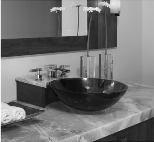
Figure 7-28 Good spacing of faucet with a vessel sink. (Photo courtesy of Mary Fisher Designs.com, Northlight Architectural Photography.com)
