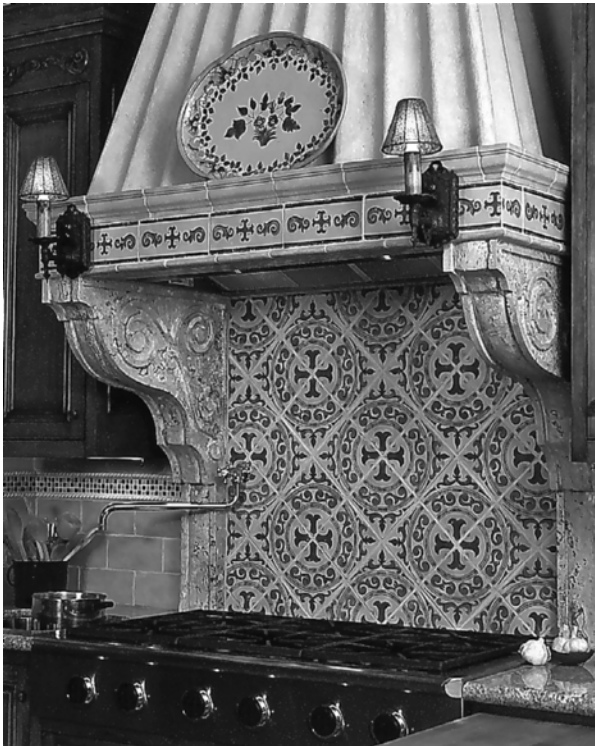
Figure 4-31 When a pot-filler faucet is planned at a range or range top along with a preparation sink, the pot filler can serve the pots at the range as well as the sink to the side. (Photo courtesy of Mary Fisher Designs.com, Northlight Architectural Photography.com)
