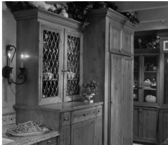
Figure 6-9 Decorative iron panels must fit door frames or vice versa. (Photo courtesy of Mary Fisher Designs.com, Northlight Architectural Photography.com)
