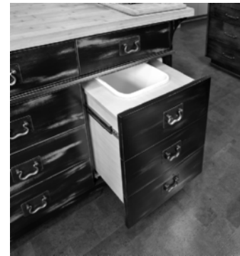
Figure 4-55 A pull-out trash container is easily accessed from the sink or cooktop. (Courtesy of Judy Svendsen, ASID, Raven Interiors/Mary Fisher Designs.com)
