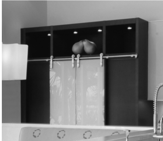
Figure 2-10 Sliding doors on an exposed track are also used on cabinetry. Consider where the door hangs when opened, whether as an entry door or a cabinet door. (Photo courtesy of Downsview Kitchens, www.downsviewkitchens.com )
