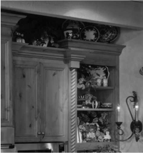
Figure 6-11 When upper cabinets vary in height, the crown molding must return to a cabinet side or face frame. If you select a frameless style of cabinet, the termination point of the crown must be altered or a filler must be installed to terminate the crown molding. (Photo courtesy of Mary Fisher Designs.com, Northlight Architectural Photography.com)
