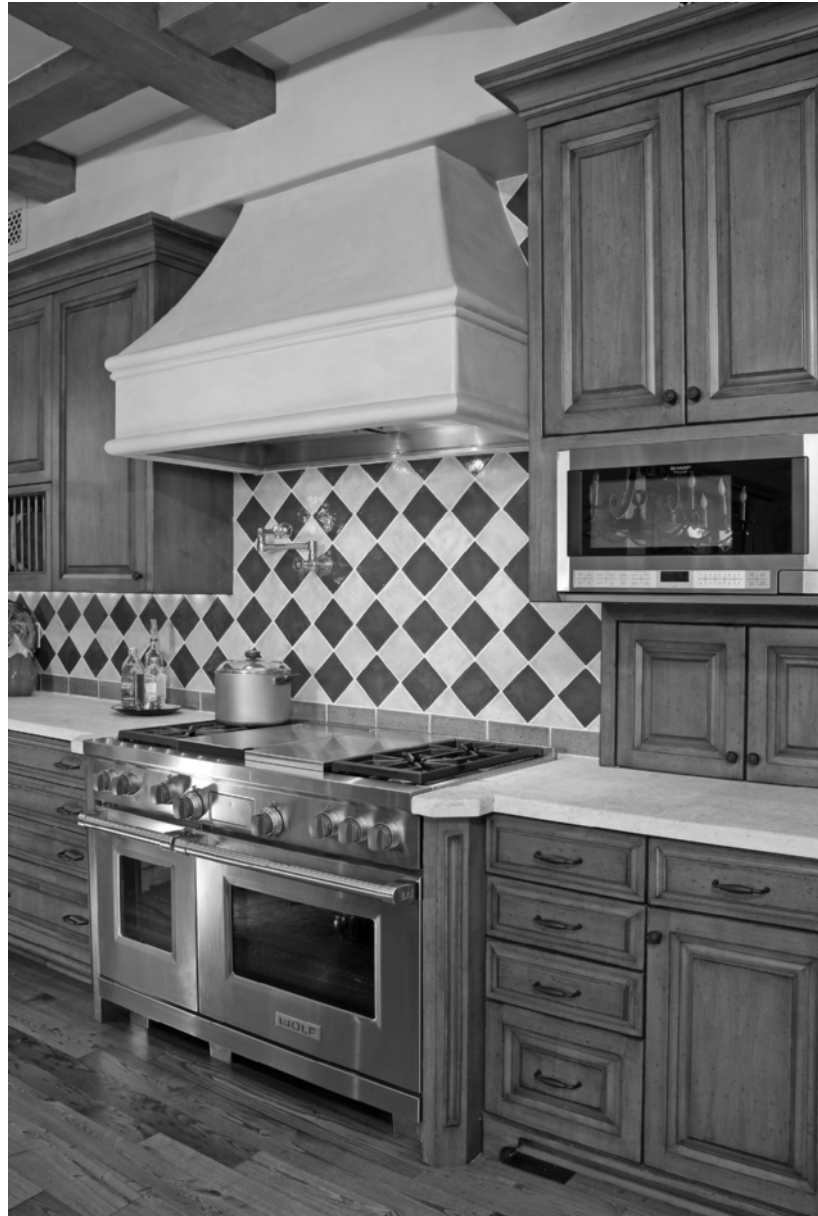
Figure 10-1 Custom hood liner vents professional style range. (Photo courtesy of Mary Fisher Designs.com, Northlight Architectural Photography.com)
