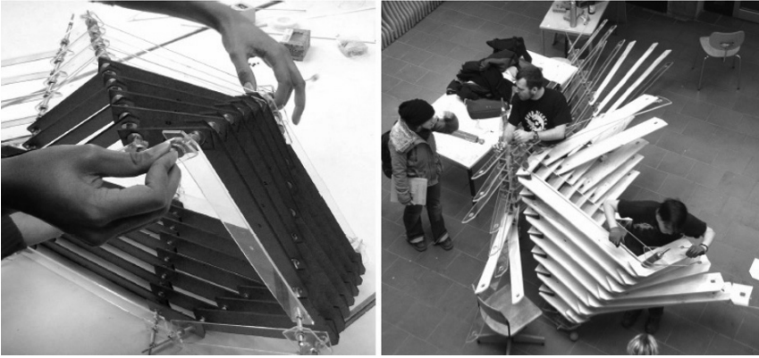
Fig. 9. Physical model in scale 1:5 (left) and pre-assembly of segmented parts (right). Photos courtesy of Technische Universität Darmstadt
