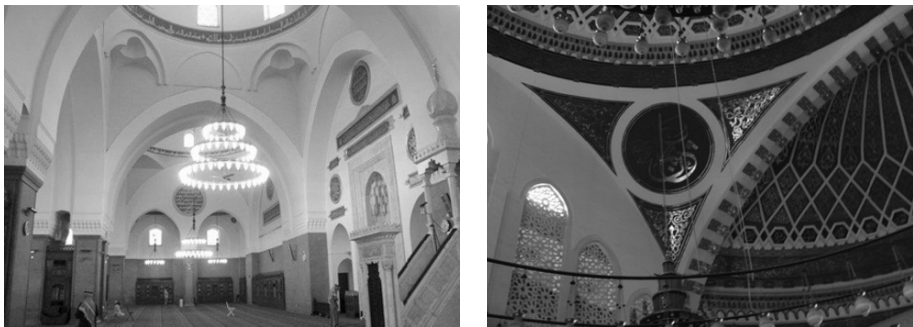
Fig. 26. Although the various methods available now to support a dome, the squinsches and pendentives are still favorable for the architects of the Islamic world. a, (left) Spherical-pointed vault squinsches in Qeba'a Masjid, Almadena Almonawara, Saudi Arabia; b, (right) pendentives in Elhosaree Masjid, 6th of October City, Egypt
