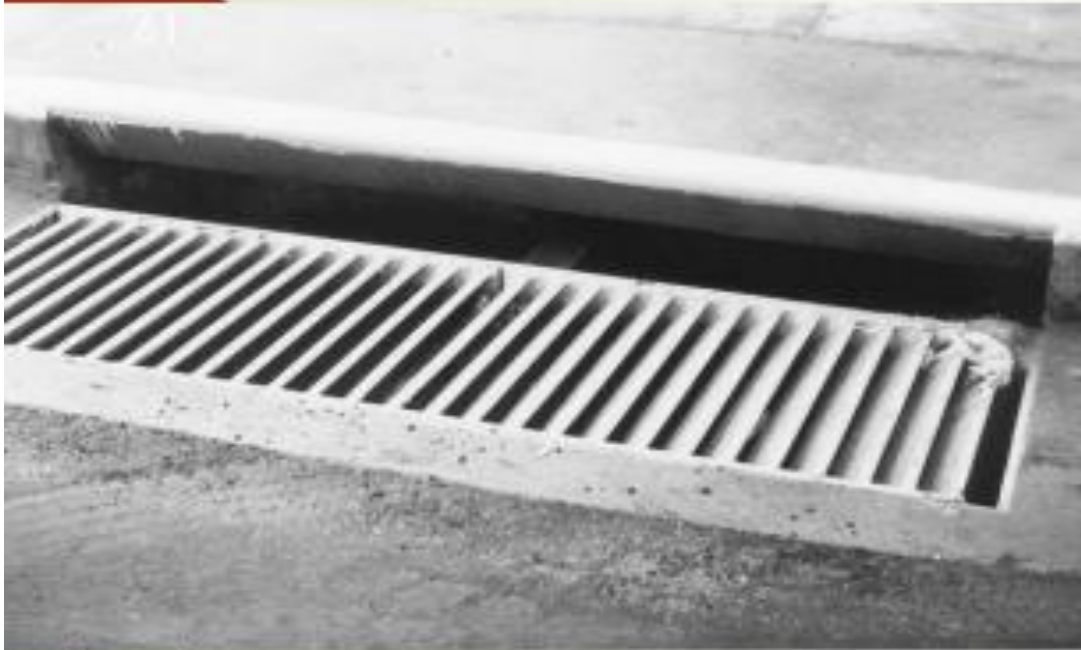
Fig 2.12 Combination inlet
