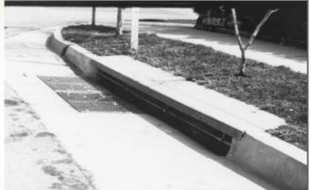
Fig 2.12 Combination inlet
