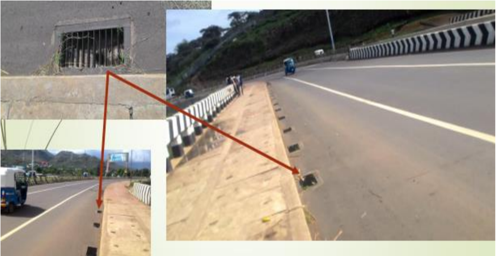
Fig 2.7 grate inlet at Kulfo bridge
