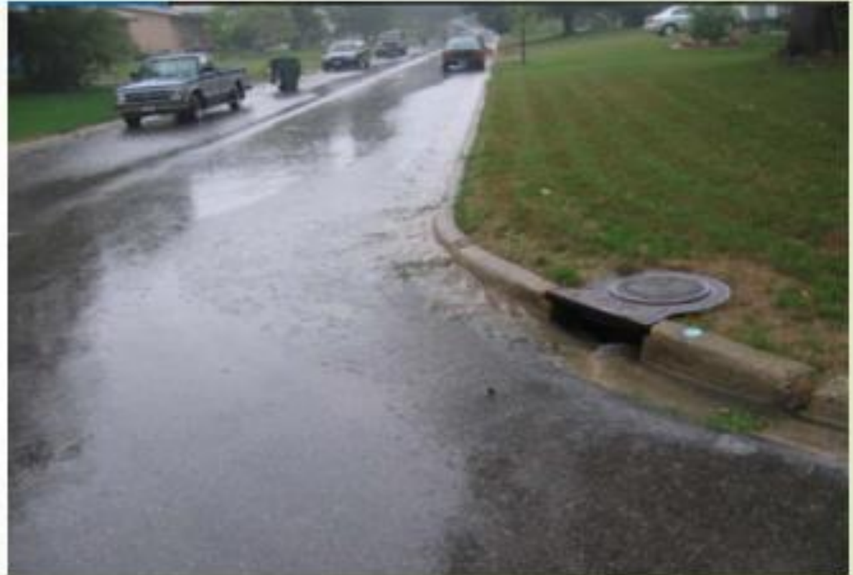
Fig 2.10 Curb opening inlet
