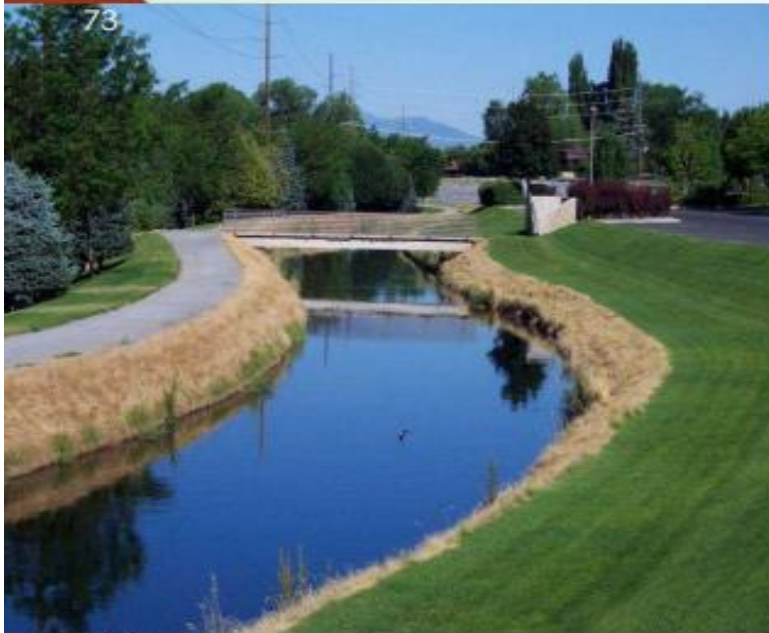
Fig 2.14 (a) and (b) large canals (i.e., typical examples of major storm drainage systems)
