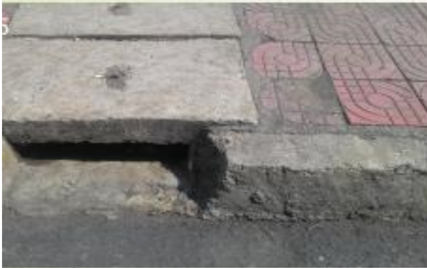
Fig 2.10 Curb opening inlet
