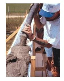
Concrete pump (through pipe)
