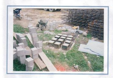
Concrete cube samples from site are tested for their actual strength and compared with design strength. Max compressive strength
