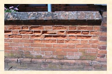
Highly absorptive bricks can cause efflorescence.
