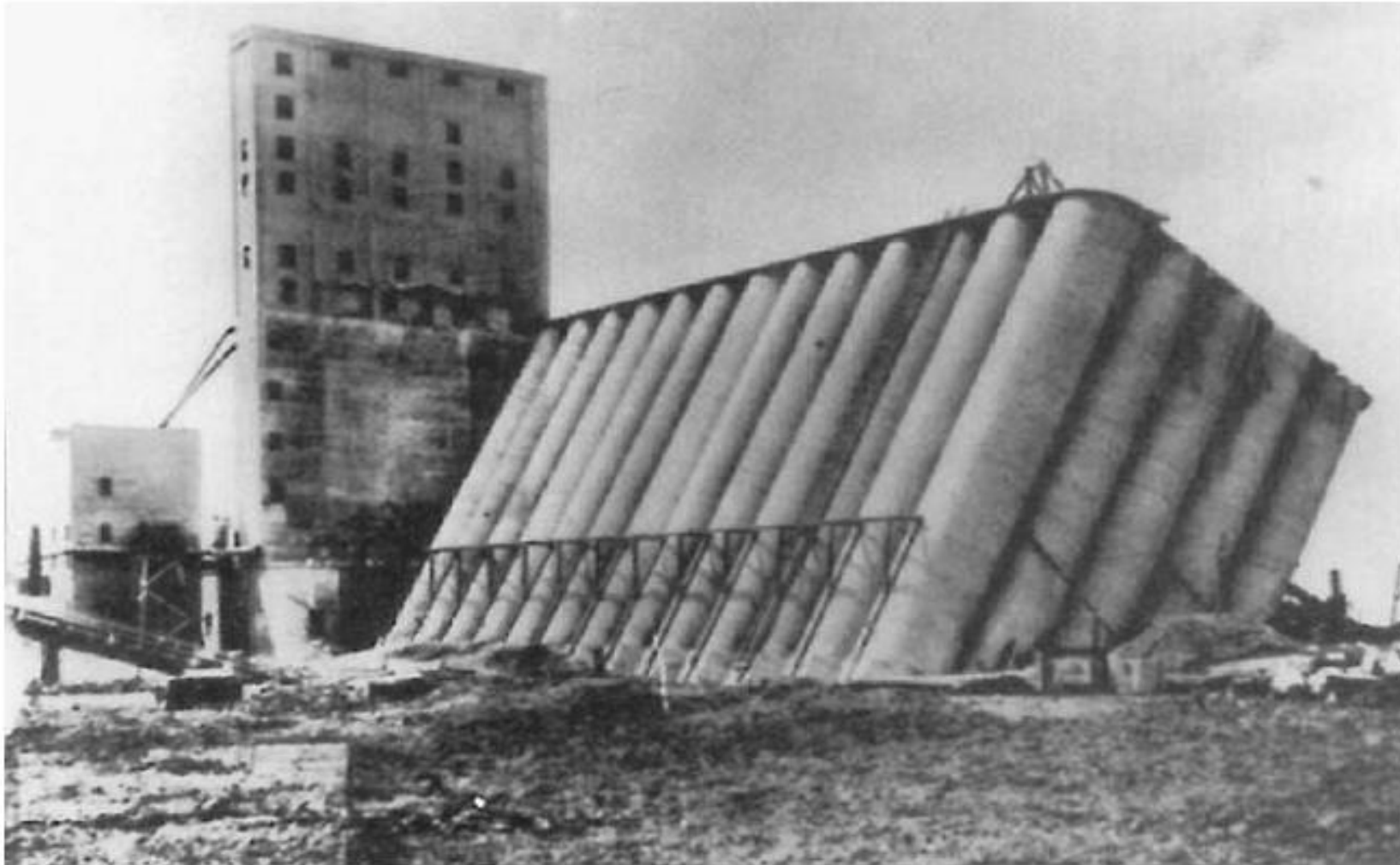
FIGURE 6.4 Transcona grain elevator failure.
