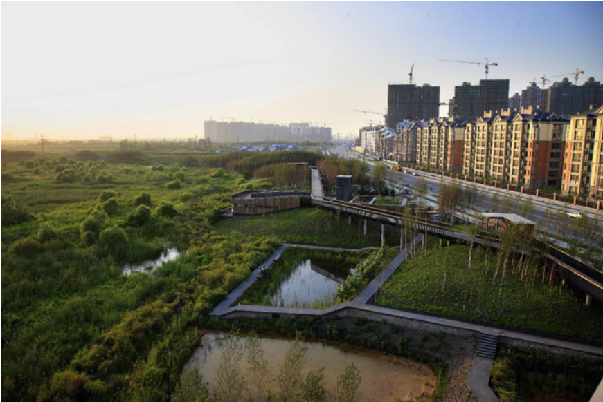
Fig. 13 Qunli Storm-water Park: cut-and-fill to create an outer ring of mounds and ponds acting as a stormwater filtrating and cleansing buffer zone for the core wetland, and a transition between nature and city (Photo Yu)
