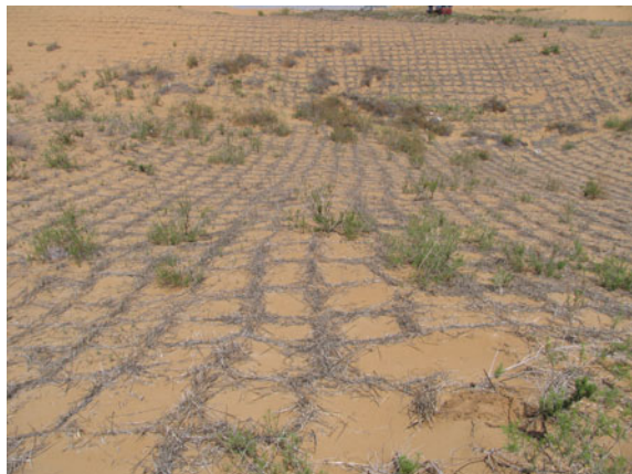
Fig. 4 A framework of sand barriers in the Shabotou sand dunes
