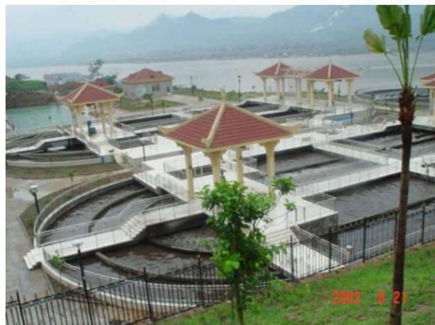
Fengdu Sewage Treatment Plant
