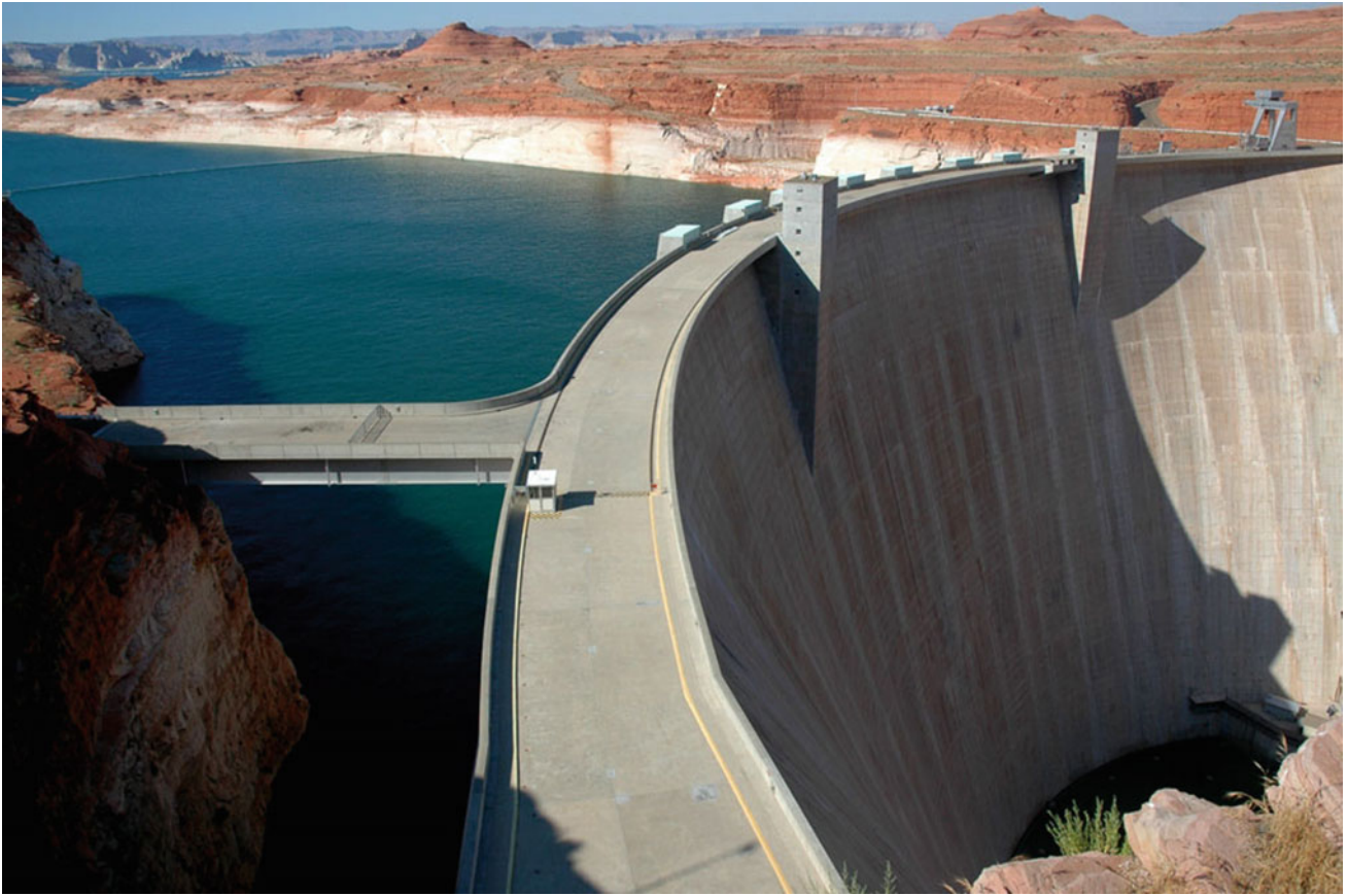
Glen Canyon Dam
