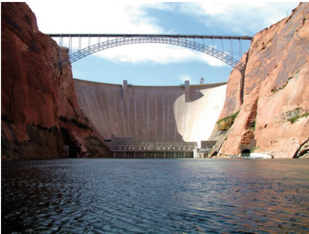
Front view of the Glen Canyon Dam
