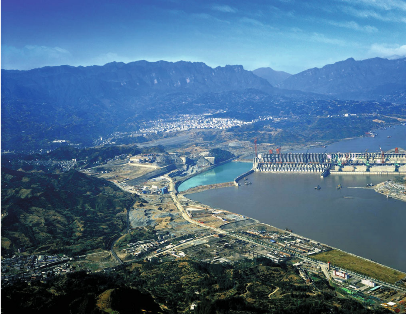
Panoramic view of the TGP in construction
