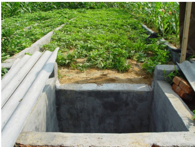
A brick-and-cement sand deposit pit is build below each runoff plot, which measures 1 m 3 in volume, 1 m deep and has a cover to prevent rainwater from falling directly into the pit. The picture shows the runoff plot (yellow soil, vegetable-potato intercropping, 15° in gradient) at Longtanping Village, Taipingxi Town, Yiling District of Yichang City. Photo by Huang Zhenli
