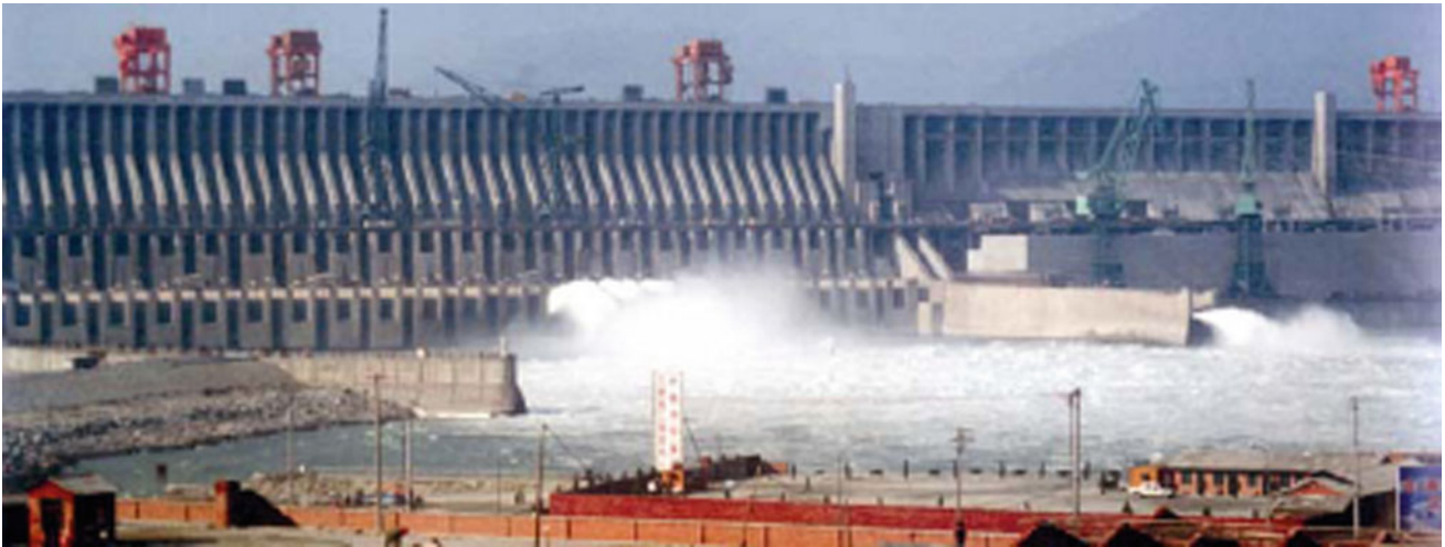
Gas oversaturation appeared in part of the downstream area in June, 2003 when the dam released water, causing significant fish biological effect
