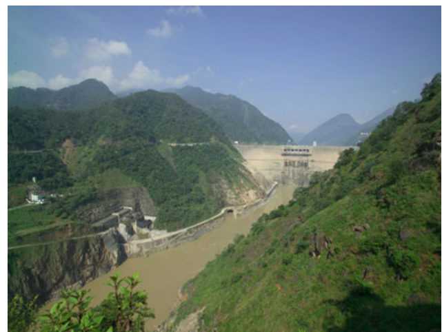
Double-arch dam at Ertan of the Yalong River (By courtesy of the Ertan Development Corporation)
