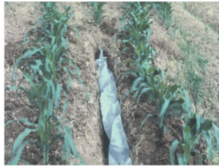
Film water blocking wall experiment at Lishu Village, town of Changling, Wanzhou district (May 1999)
