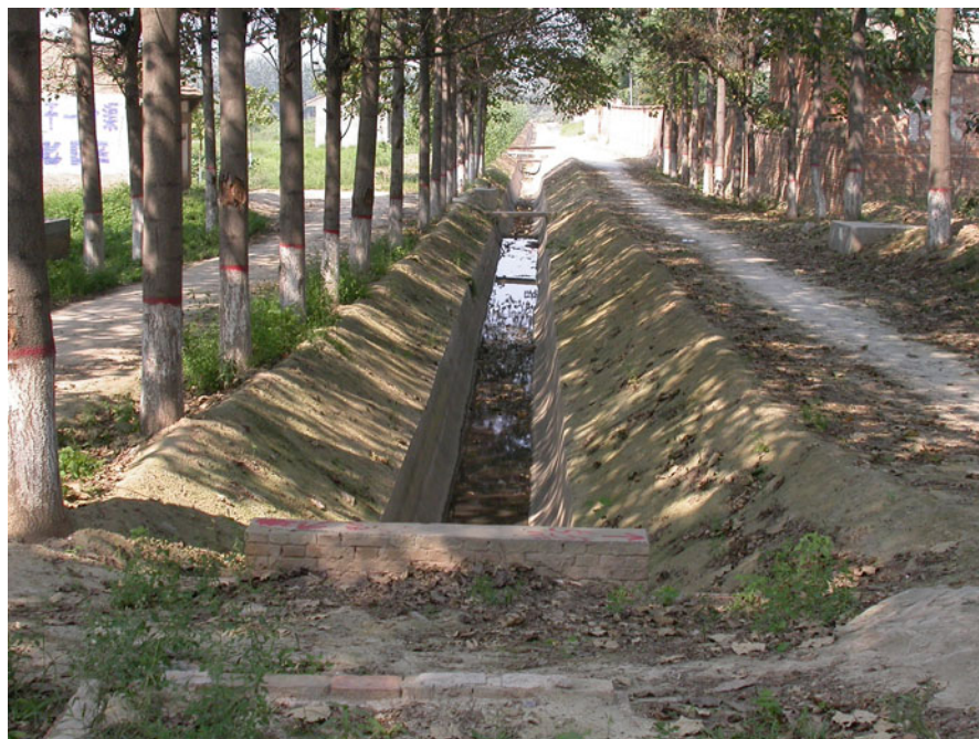
Fig. 7.7 Luohui irrigation district, secondary water channel on Luodong block central main channel
