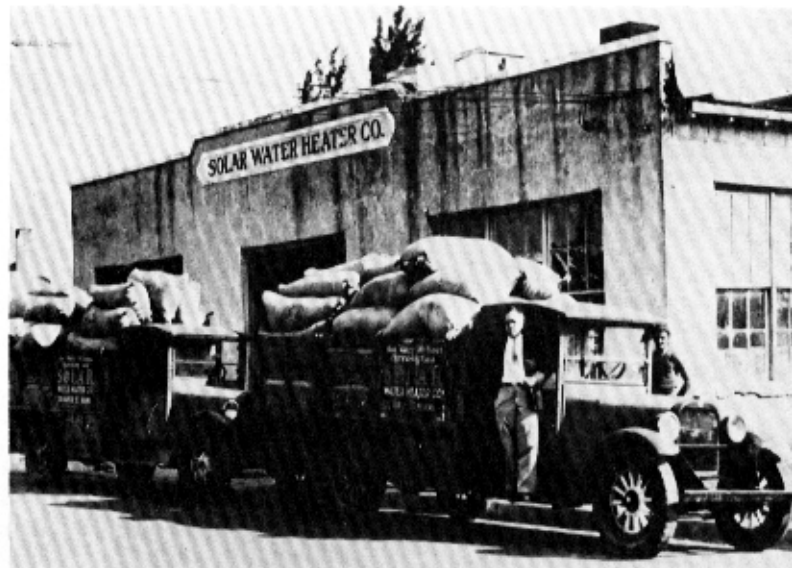
Exterior view of the Solar Water Heater Company in Miami, 1924. The company trucks are carrying large bags of cork insulation.
