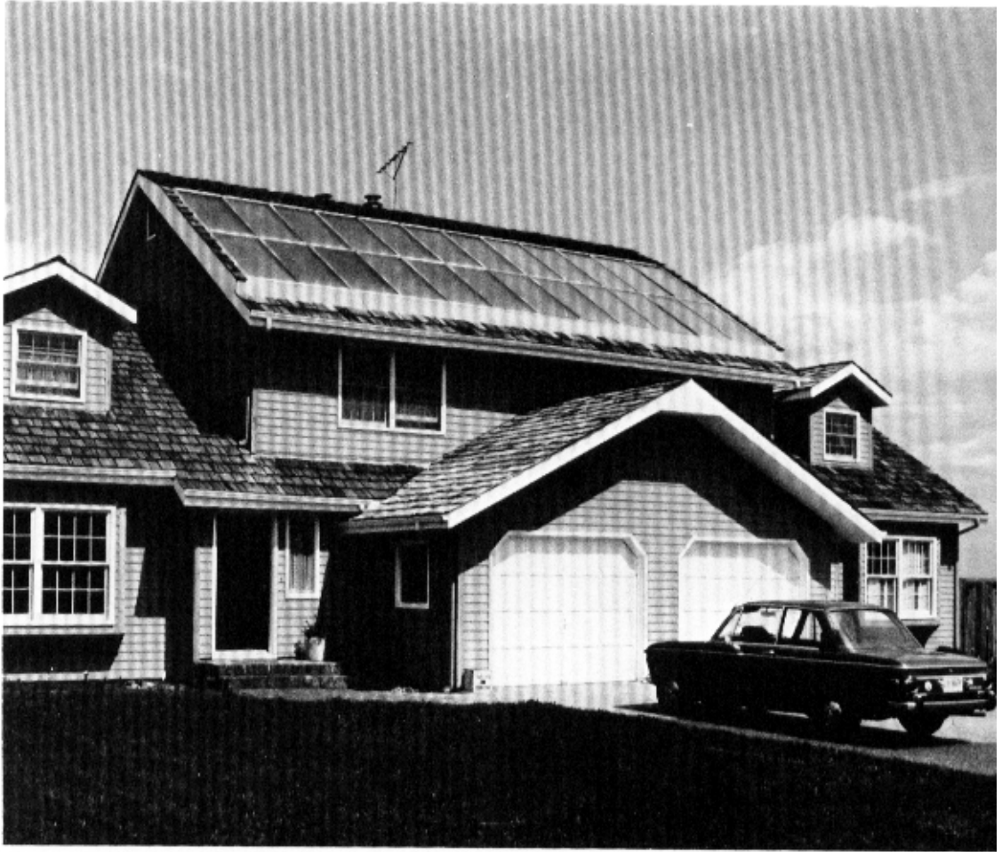
Solaron collectors heat this duplex home in Fort Collins, Colorado.
