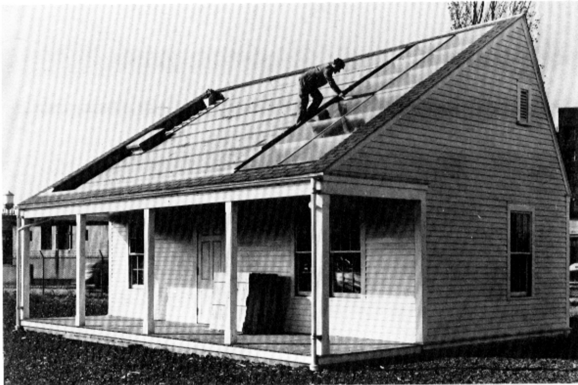
A workman installs flat-plate collectors on the first M.I.T. solar house, 1939.
