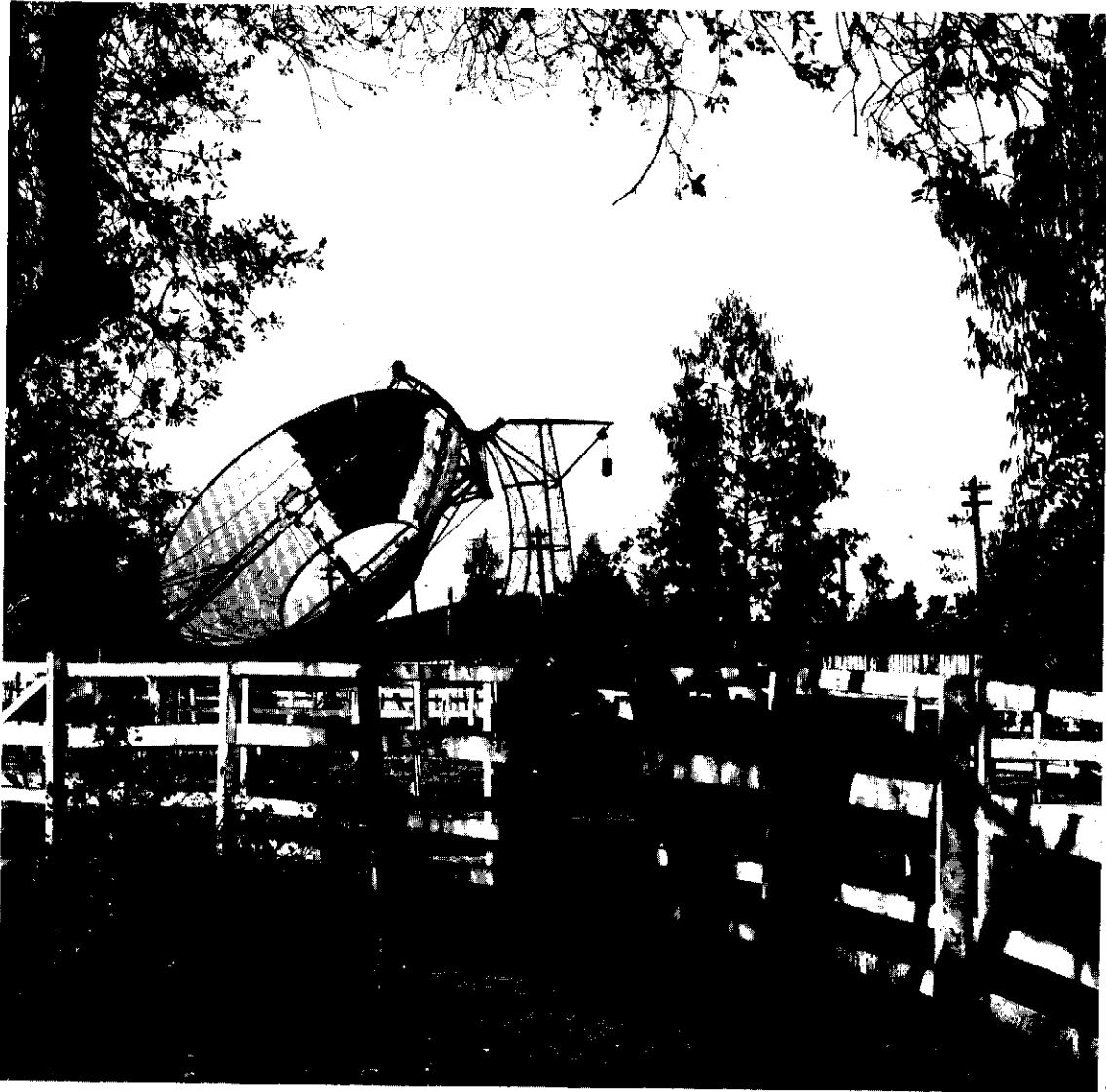
1 The Pasadena sun motor in operation. Notice the glistening white boiler and the steam escaping from a relief valve.
