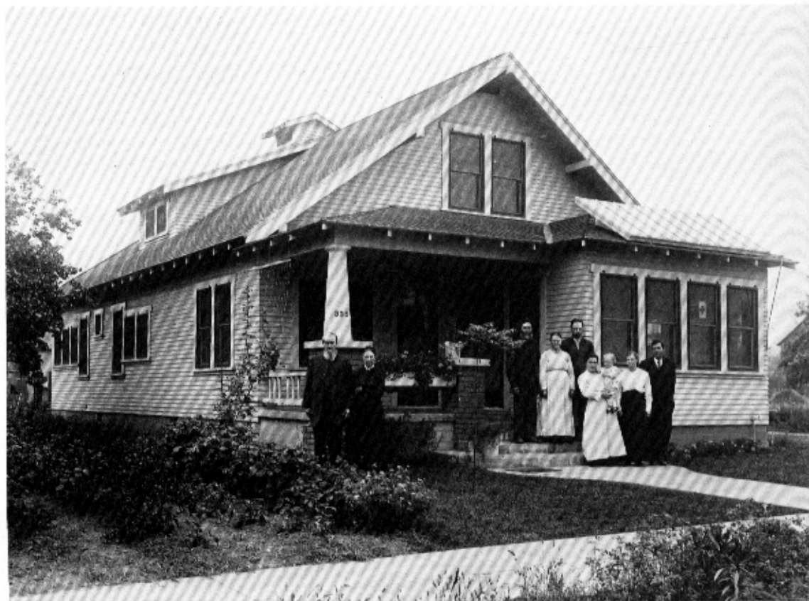
This Pomona Valley, California, family had a Day and Night solar water heater on the roof of their house in 1911.
