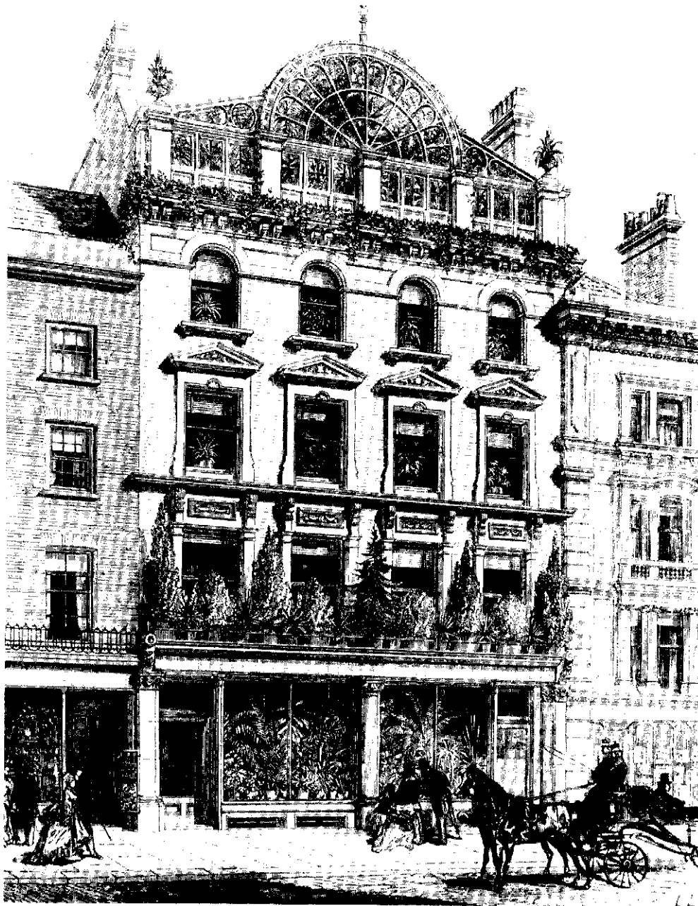
Large glass windows on the south side helped plants flourish in this London setting. A rooftop greenhouse provided further growing space.
