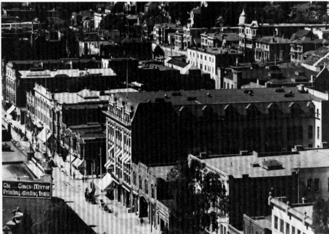
Six Improved Climax solar water heaters atop an office building in downtown Los Angeles, 1907. Close-up (top) provides a better look.
