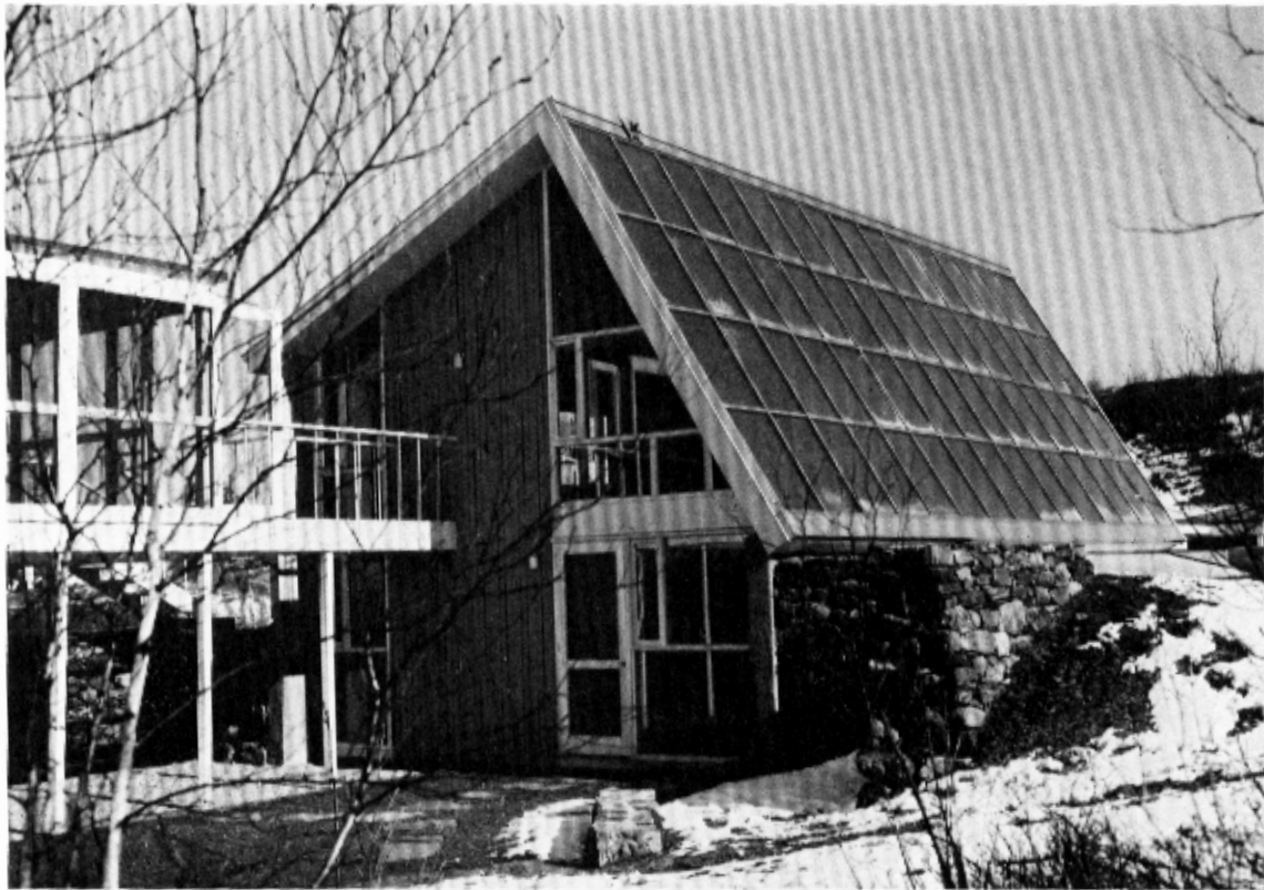
Southwest view of M.I.T.'s fourth solar house in Lexington, Massachusetts. Planned as a prototype for mass construction, it obtained half of its winter heat from the sun.
