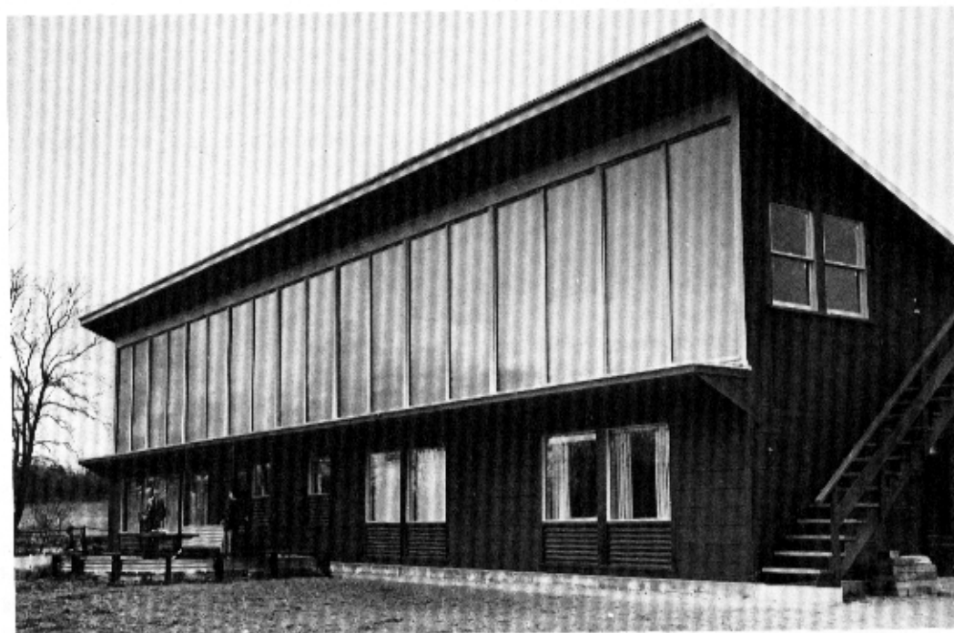
South face of the Dover house, with the Nemethy family gathered in front. Solar air-heating collectors spanned the entire second-story wall.
