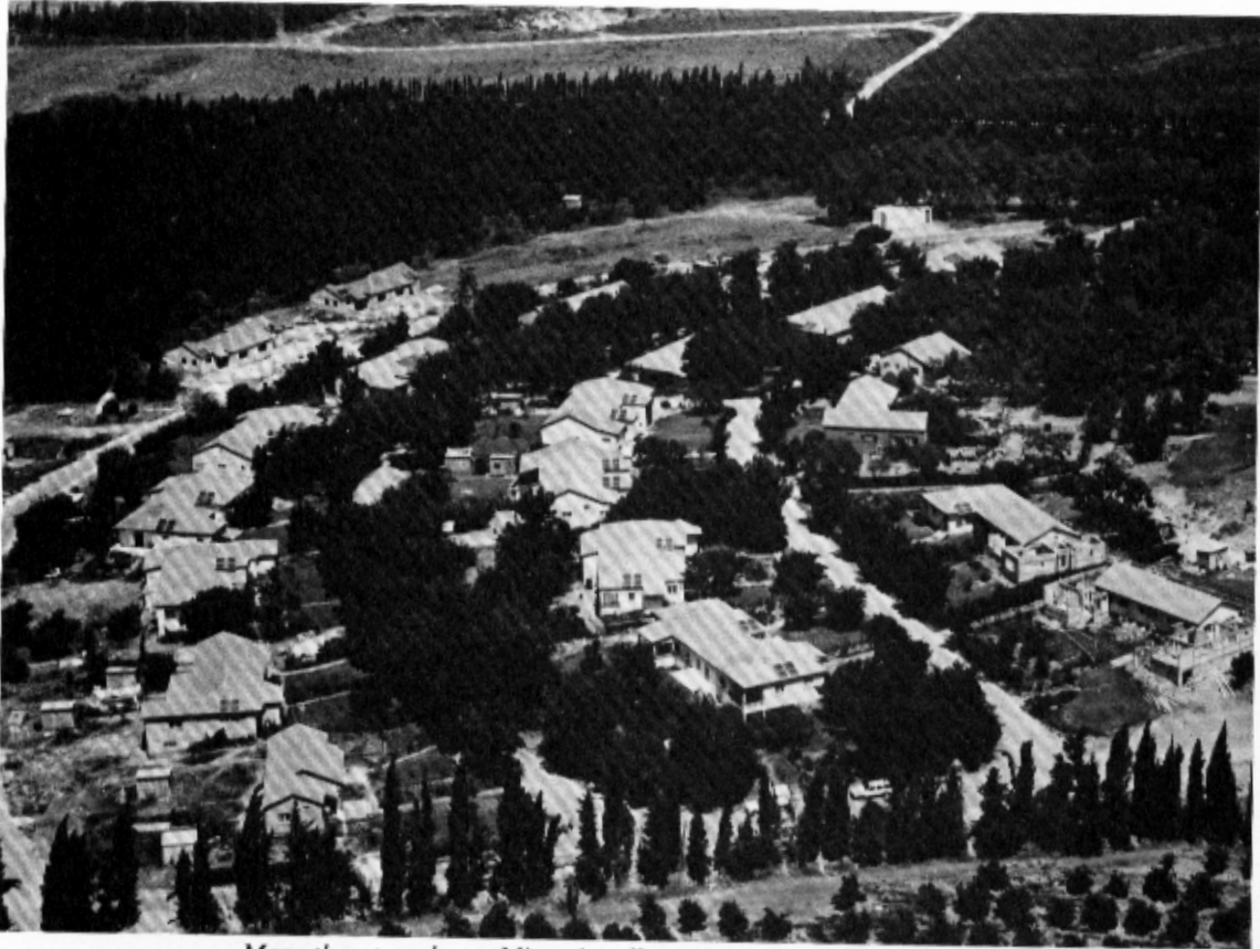
More than two dozen Miromit collectors can be seen on the roofs of these dwellings at Benai Hadarom, an Israeli kibbutz near Tel Aviv.
