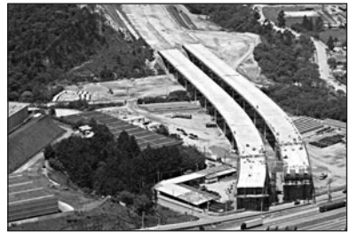
Fig. 14-7. Works of the South Segment of the Rodoanel Mário Covas
