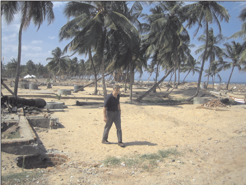
Figure 2. Photograph of the coastal area near Maruthumunai, Sri Lanka, showing the near complete destruction of homes along the coast. The photographer is standing about 150 m from the coastline, and it was reported to the team that the maximum wave height at this site reached high into the palm trees shown in the background. Note the high density of domestic open dug wells (typically short vertical circular structures), many of which were not destroyed by the wave but were inundated and flooded by seawater and debris
