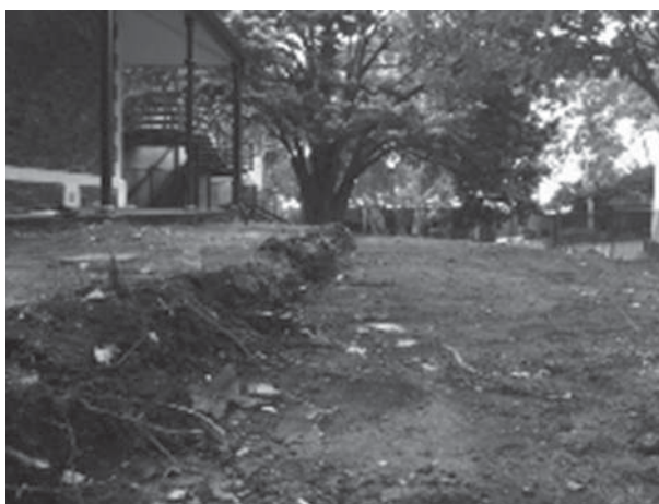
The excavation begins Rostrevor College Junior School
