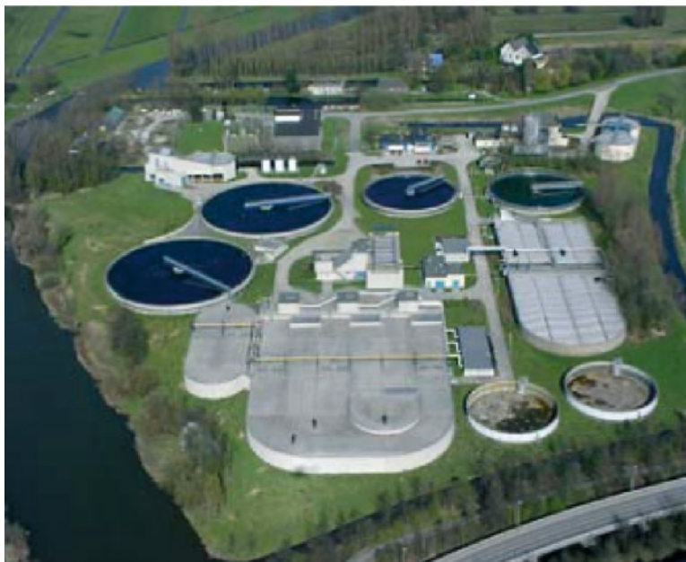
Fig. 5.4 Wastewater treatment plant, Kortenoord. Source: Water Board Schieland en de Krimpenerwaard
