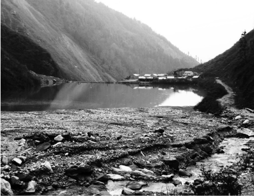
Fig. 19.3 An earthquake-generated landslide-dammed lake from the 2008 Wenchuan earthquake. The dam has been hardened with concrete and the outflow is controlled to prevent erosion of the dam and outburst flooding. The presence of the lake, however, carries the threat of a future landslide-generated flood overtopping the dam (James Gardner)
