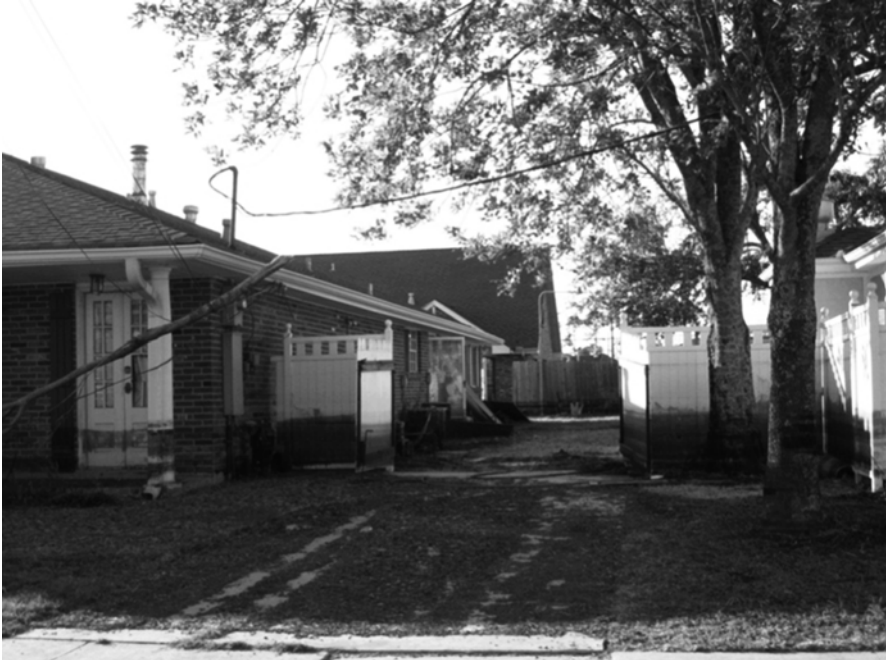
Fig. 23.1 One of more than 1,800 homes in Chalmette, Louisiana, affected by floods and an oil release from a neighboring refinery following Hurricane Katrina in 2005
