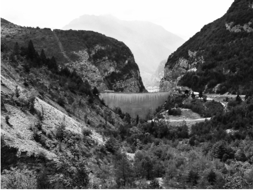
Fig. 19.6 The Vaiont Dam in the Italian Alps, now decommissioned as a hydro-electric facility following the 1963 landslide (deposit shown to the left of the photo), impact wave and flood disaster in the Piave valley. The photo is taken from the reservoir area overlooking the dam to the narrow opening to the Piave River valley and the city of Longarone (James Gardner)
