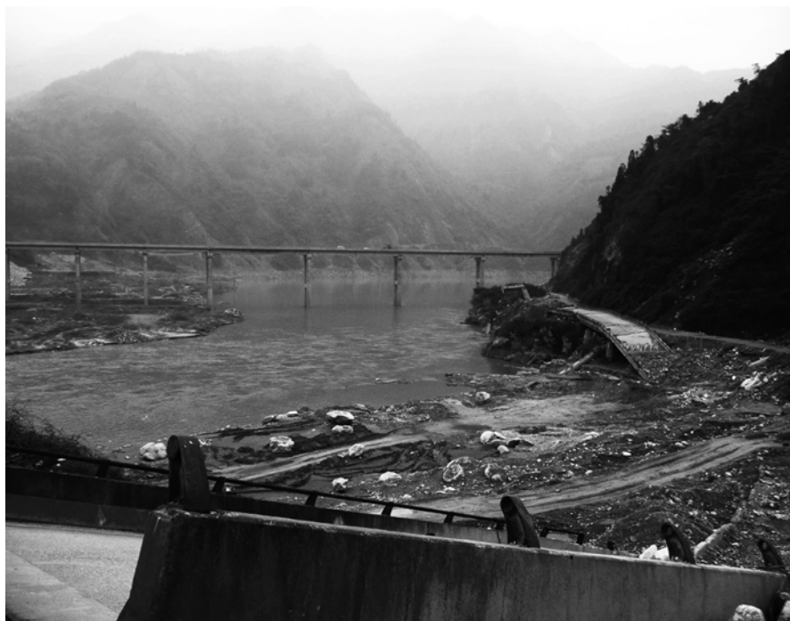
Fig. 19.2 The Minjiang valley near Yingxiu, Sichuan, showing the destruction of a national highway by the 2008 Wenchuan earthquake and landslides and 2010 debris flows. The bridge in the background carries the new route of the highway and was constructed within months of the earthquake (James Gardner)
