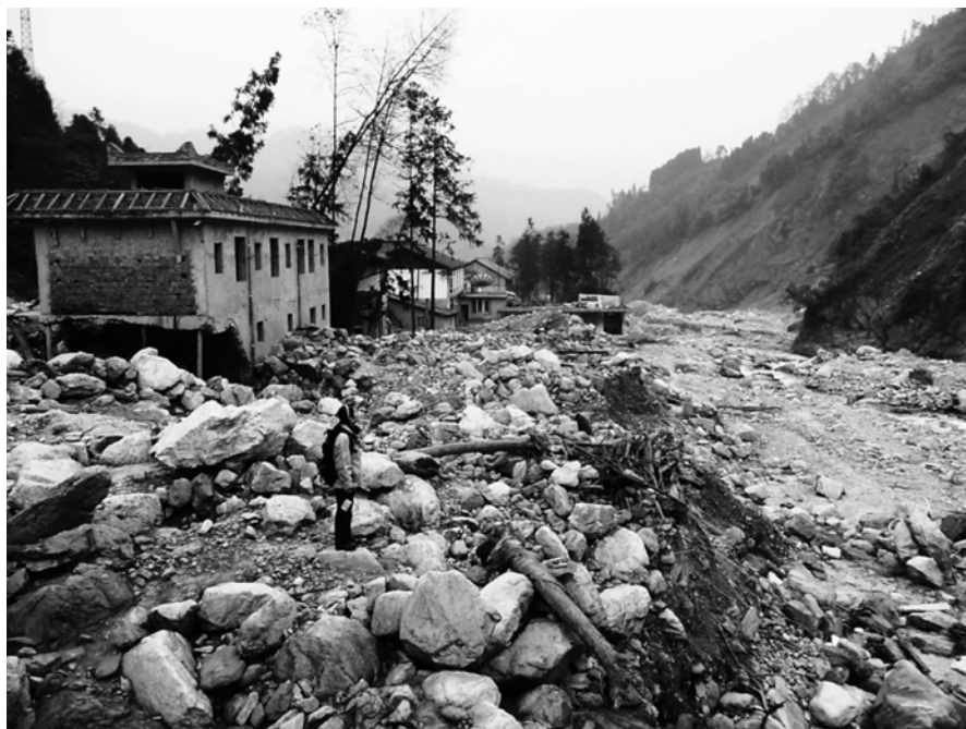
Fig. 19.4 2010 debris flow destruction, by earthquake and landslide debris, of newly (post-2008 earthquake) constructed and reconstructed hotels and shops in the Longxijiang valley, Sichuan, China (James Gardner)
