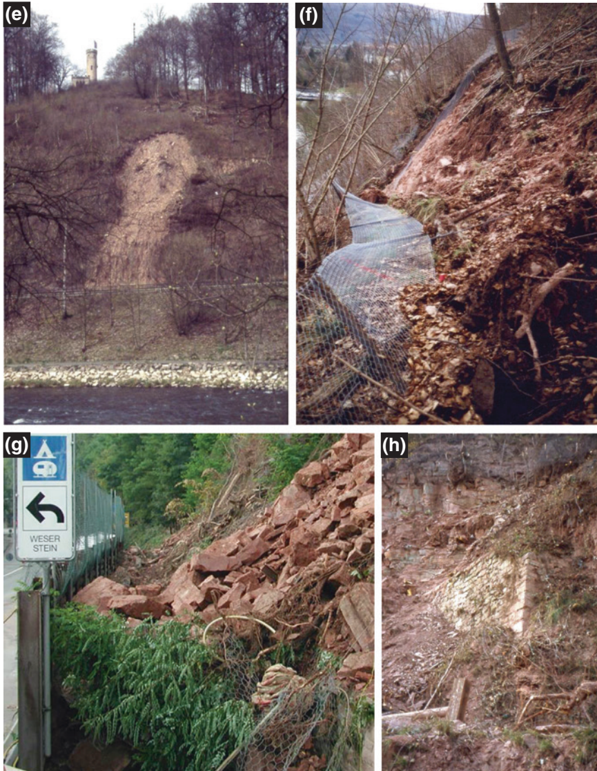
About 30 landslide events occurred during the 20th century with clusters in 1924–1926, 1961, 1970, 1974, 1994, and 1999–2001 (e). Implementation of low-cost mitigation measures (catch fence, rockfall drapery, etc.) in response to these damage events, but hazard mitigation was usually undersized and failed under stress, therefore not enabling effective risk reduction (f,g,h).
