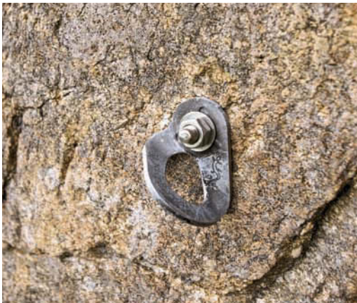
Figure 8.11 An example of a good and reliable bolt.
