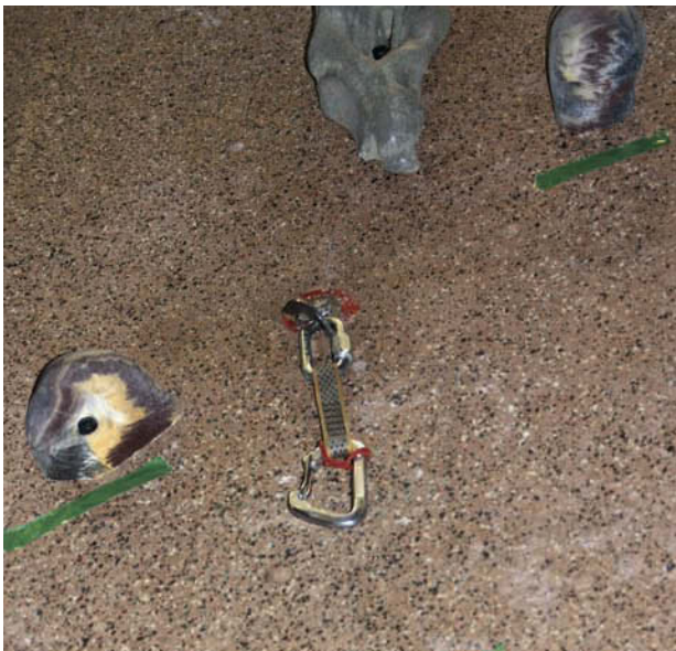
Figure 3.13 Lead anchors can only be used in indoor climbing facilities that have load-bearing framing.
