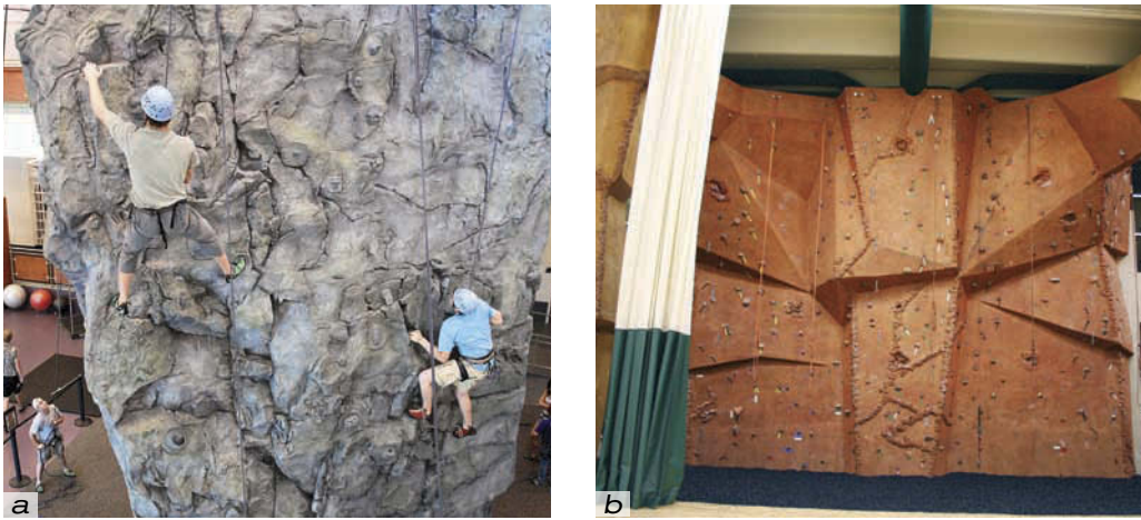
Figure 3.3 Walls with surfaces made of (a) glass fiber reinforced concrete and (b) wood covered in concrete are commonly found at both universities and commercial climbing gyms.
