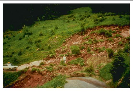
**Photo 2.15** In case an object is situated underneath a landslide, negative consequences are caused by the dynamic impact of the moving mass and burial with landslide deposits. This photo shows a small landslide that blocked a road near Montagnier, Canton du
