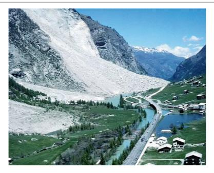
**Photo 2.7** Screes do not infrequently aggravate the construction and maintenance of diverse linear objects, for example, auto roads and railroads, pipelines, and power lines. Their impacts are exerted both through dynamic impact of fragmental products
