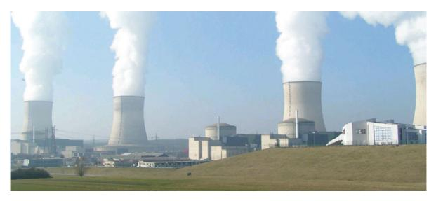
**Photo 8.9** The thermal pollution from nuclear power plants is greater than that from thermal power stations. Heat is released by NPPs through condensation systems with cooling water and
