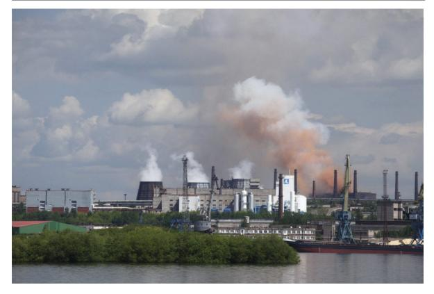
**Photo 9.10** Gaseous pollutants of ferrous metallurgy enterprises include the following substances: (1) sulphur dioxide related to the presence of sulphur in fuels or ores, (2) nitrogen oxides emitted to the atmosphere as combustion products, (3)
