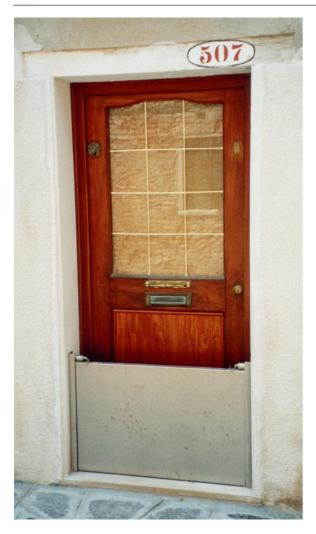
**Photo 4.8** Wind-induced surges are typical of Venice, Italy. The photo shows a house door with an additional hermetic barrier, which protects the house from seawater (Photo credit: Lee Bosher, Loughborough University, United Kingdom, August 2003)
