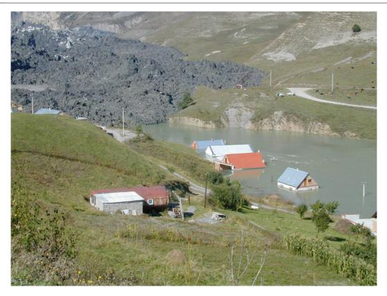
**Photo 4.40** The impact of the Kolka surging glacier on dwellings during the surge of 20 September 2002 resulted in both destruction of buildings due to dynamic impact of ice and debris and their further inundation by melted ice. The photo shows a
