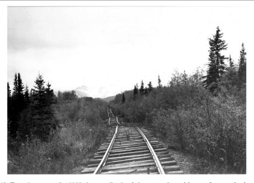
**Photo 1.19** Thermokarst poses a formidable threat to railroad maintenance. The photo illustrates the numerous deformations of the Northwestern Railway near Strelna, 75 miles northeast of Valdez, Alaska (United States). The thermal equilibrium of the fine-grained sediments underlying the roadbed was disrupted
