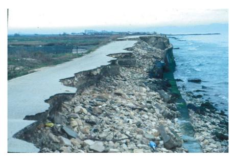
**Photo 2.42** The effects of abrasion on engineering structures are caused by the undercutting of bank slopes and their subsequent collapse. This road on the coast of the Adriatic Sea,
