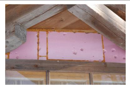
**Photo 5.110** Birds, to a certain degree, complicate the maintenance of residential structures. For example, they withdraw an oakum from blockhouse slots for nest construction and contaminate walls, windows and other structures with their droppings The damage done by Eurasian green
