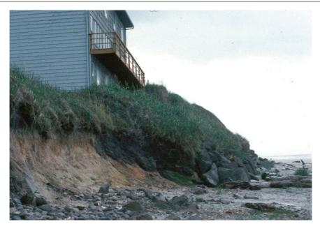
**Photo 2.41** The coast retrogression rate in the case of abrasion depends on many factors (e.g. strength and hydro-resistance of rocks, depth of the coastal zone, and prevailing wind directions) and varies within a wide range: from several centimetres to
