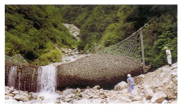
**Photo 2.23** Protective measures against mudflows are varied. One of them is installation of flexible mesh barriers. The photo shows a flexible mesh barrier in the area of Aobandani, Japan, to protect against debris flow. It is 20 m long and 4 m high and is
