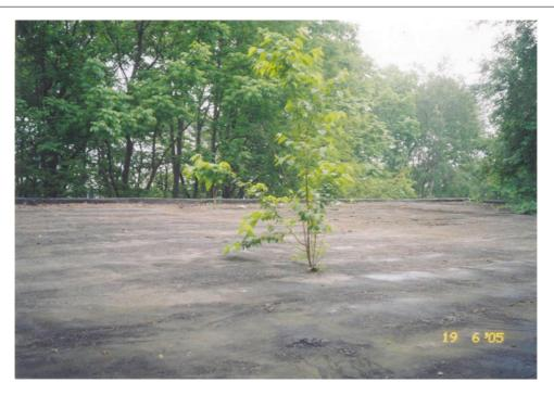
**Photo 5.106** Devastating effects of plants may be due to things such as wedging by their roots, creating conditions for penetration of moisture and destruction of binding materials with root
