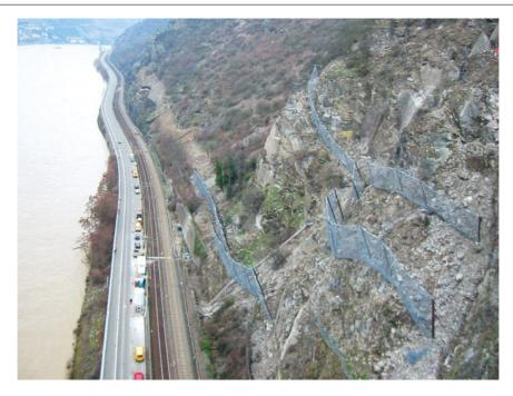
**Photo 2.4** Mitigation measures against rockfalls are usually costly. The most exposed sites are typically protected by special flexible anti-rockfall barriers. Elements of a particular protective system are chosen based upon the presumable power of a
