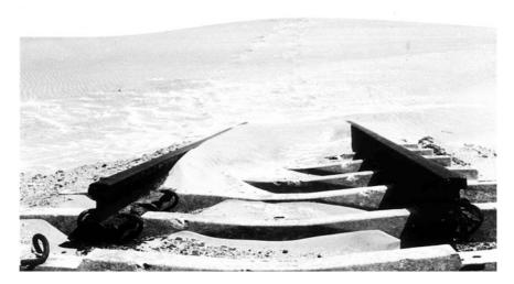
**Photo 2.29** Dunes encroaching at speeds of tens of metres per year many times blocked the 200 km long railroad between Walvisbaai and Swakopmund, Namibia. The attempts to stabilize the movement of dunes by means of
