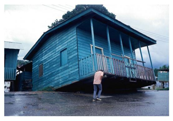
**Photo 3.33** In many cases, small houses are damaged by strong winds directly. The photo shows a house in Honduras that was blown off its foundation by Hurricane 'Fifi'. (Photo credit: UNESCO, M. Ginies, 1974)
