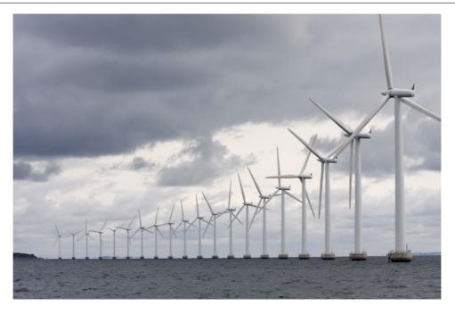
**Photo 8.15** According to where they are placed, the following types of wind power plants can be identified: (1) ground (wind turbines are usually installed in the hills); (2) coastal, or onshore (a small distance from the sea coast); (3) offshore (constructed at
