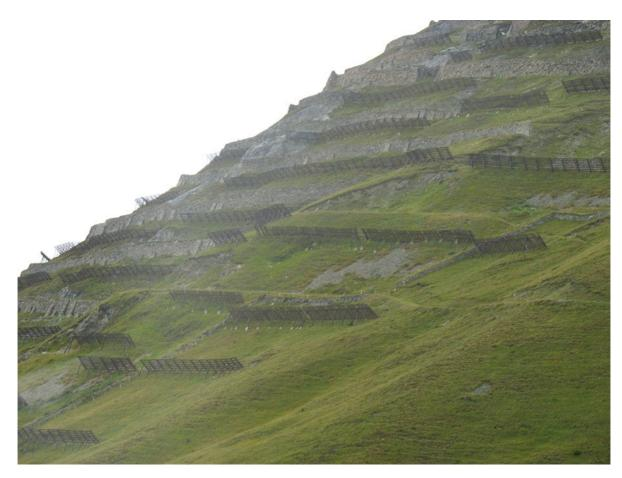
**Photo 2.11** There are many ways to protect objects and people from avalanches. One of them is erecting snow-stabilizing barriers. The increase in roughness of the slope surface helps stabilize the snow blanket and prevents avalanches from passing. The
