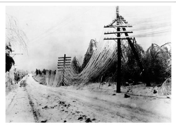
**Photo 3.44** Ice-up destroys communication and power lines. The weight of ice crusts can reach 86 kg/m. The photo shows a telephone line covered with ice in the United States (Photo credit: U.S. National Oceanic and Atmospheric Administration)
