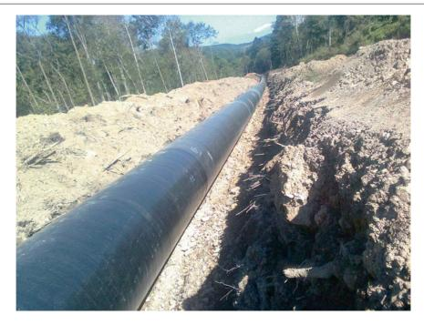
**Photo 12.10** The next stages in building a pipeline over land are: (3) making ditches; (4) laying the pipes along the route of the pipeline; (5) pipe bending; (6) welding; (7) wrapping the pipes with polymeric bands; (8) applying an insulating coating; (9) installing cathodic corrosion protection systems; (10) laying
