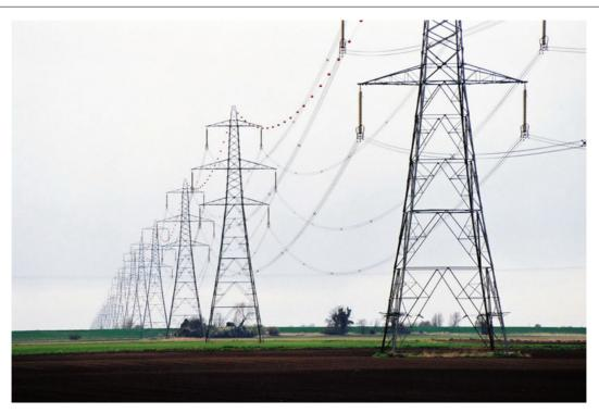
**Photo 8.28** An area with a radius of 2 m around towers is allotted for use by a power transmission line on a permanent basis. This situation affects agriculture to the greatest extent. The disordered arrangement of power transmission and telephone lines
