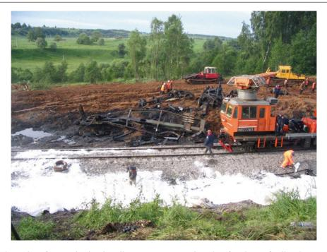
**Photo 12.8** The scales of contamination in rail transport increase many times in case of emergency. As a result of a derailment of a freight train on 15 June 2005, near Rzev (Tver oblast, Russia), 21 tanks with fuel oil overturned. Altogether, about 300 ton of oil products were released. Removing the
