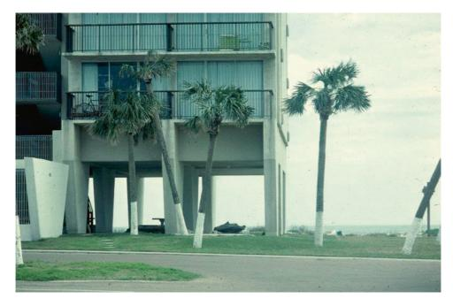
**Photo 4.31** One of the ways to protect dwellings and industrial structures from dynamic impact of waves is to make the first floors of buildings maximally open. The photo shows a house on
