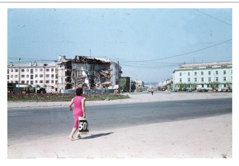
**Photo 1.18** The photo shows a wall collapse in a dwelling in Yakutsk, Russia, caused by thermokarst. Nobody was injured. To prevent such collapses, houses must be built on piles. Thereby, the air space under the house should prevent the heat impact on the frozen ground. This house was erected 'low-sitting', and for
