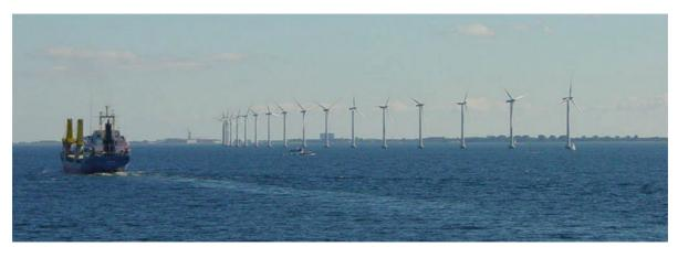
**Photo 8.16** Middelgrunden is an example of an offshore wind farm. It is in the Øresund, 3.5 km outside Copenhagen, Denmark. When it was built in 2000, it was the world's largest offshore wind farm, with 20 turbines and a capacity of 40 MW. The farm
