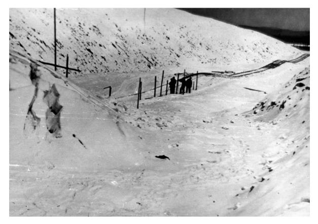
**Photo 1.17** Mounds of heaving ground do not have considerable impacts on humans since the lands where they occur are usually sparsely inhabited and poorly developed. The photo shows mounds of heaving ground on the Tynda–Zeysk section of the Baykal–Amur Railroad, Russia (Photo credit: V.S. Afanasenko, Department of Geocryology, Moscow State University, Russia)
