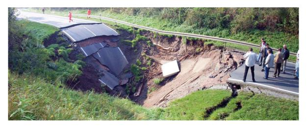
**Photo 1.29** The effects of karst on auto roads and railroads are also widespread. The photo shows damage to Road 180 due to a sinkhole in the south of Lutherstadt Eisleben, Germany, in 2001 (Photo credit: State Office for Geology and Mining, Saxony-Anhalt, Germany)
