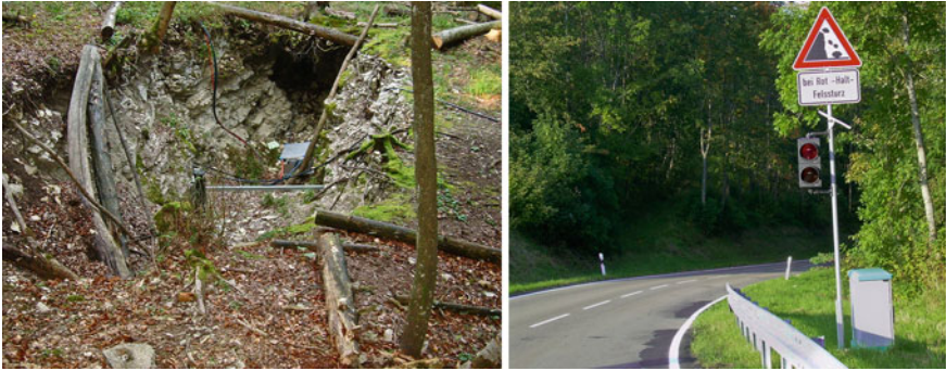
Fig. 2.10 Early warning system at Winkelgrat landslide equipped with automatic extensometers ( left ) and traffic light for road closure ( right )
