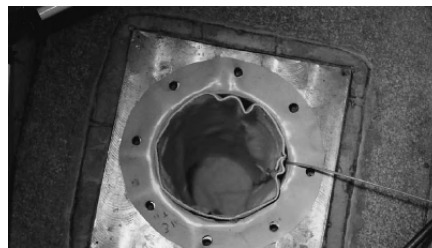
Figure 11.2. The geotextile interface and geosynthetic liner
