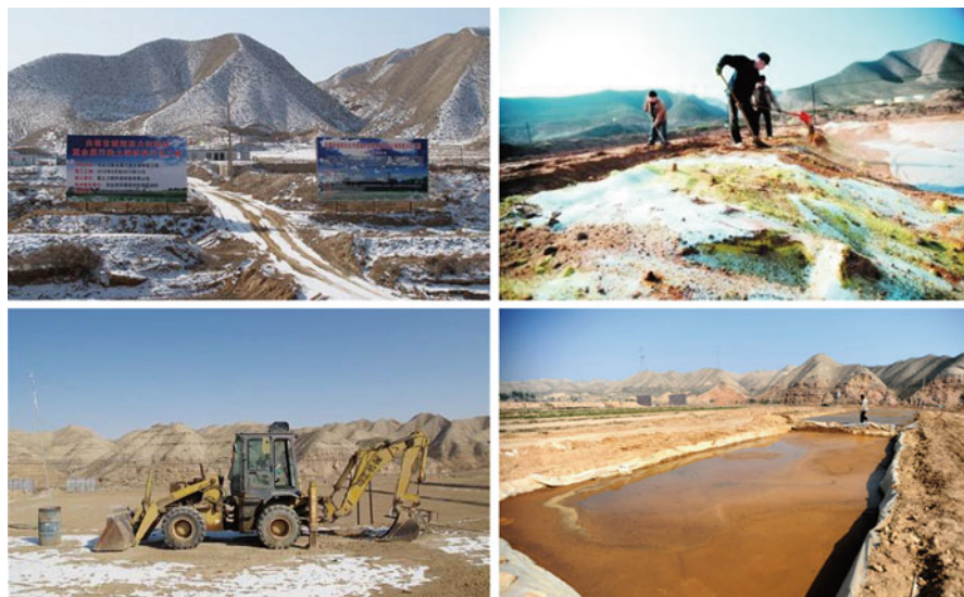
Fig. 2 A government-run soil pollution clean-up project using soil washing technique along Dongdagou in Gansu Province, northwest China
