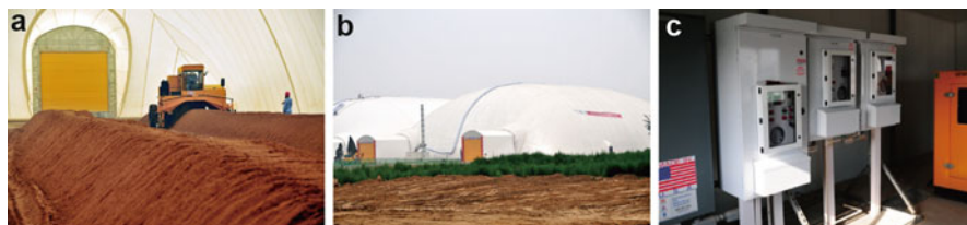
Fig. 12 Field remediation of chloride hydrocarbons by mechanical aeration. (a) Agitation. (b) Airtight shed. (c) Tail gas monitoring system
