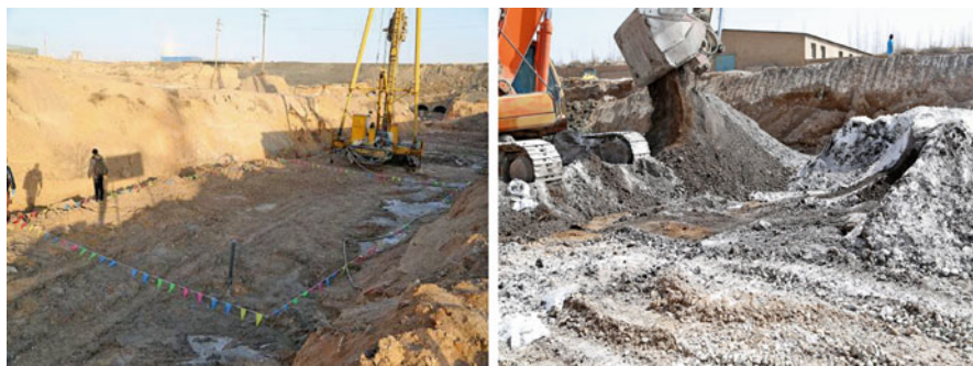
Fig. 5 Remediation project of heavy metal-contaminated industrial site in Gansu Province
