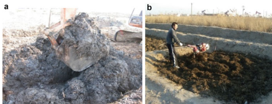
Fig. 4 Field-enhanced bioremediation of oil sludge by landfarming with the addition of straw residues. (a) Mixing the oil sludge and cotton straws. (b) Rotary tillage during landfarming treatment
