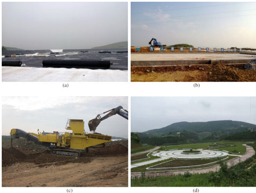
Fig. 5 Demonstration project of heavy metal-contaminated soil in Hubei province. (a) The temporary storage land for the contaminated soil (under construction). (b) The S/S treatment factory. (c) S/S process. (d) The current situation of after-treated site
