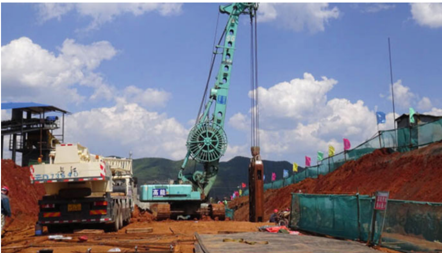
Fig. 2 Vertical barrier system construction
