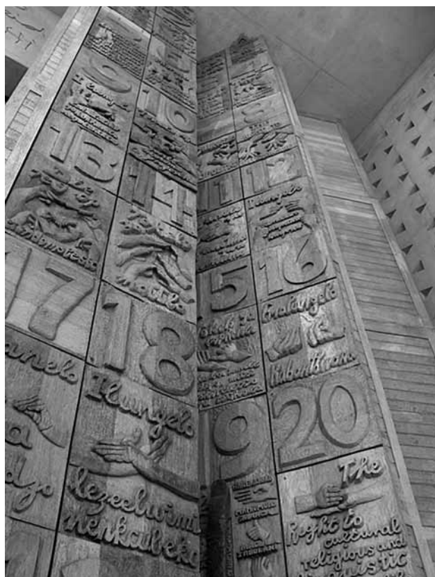
8.4 View of the doors to the Court Building (photo by David Viljoen)
