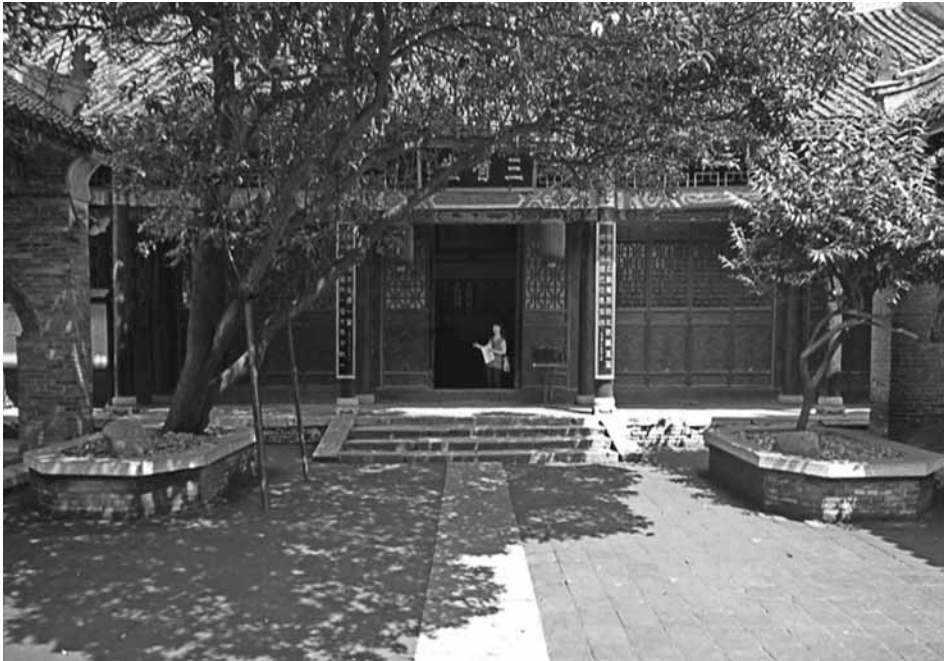
9.13 View of the courtyard of the magistrate's house leading to the final hall (photo by author)
