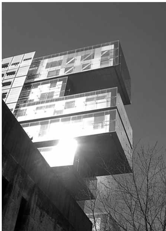
5.1 Manchester Civil Justice Centre (photo by author)
