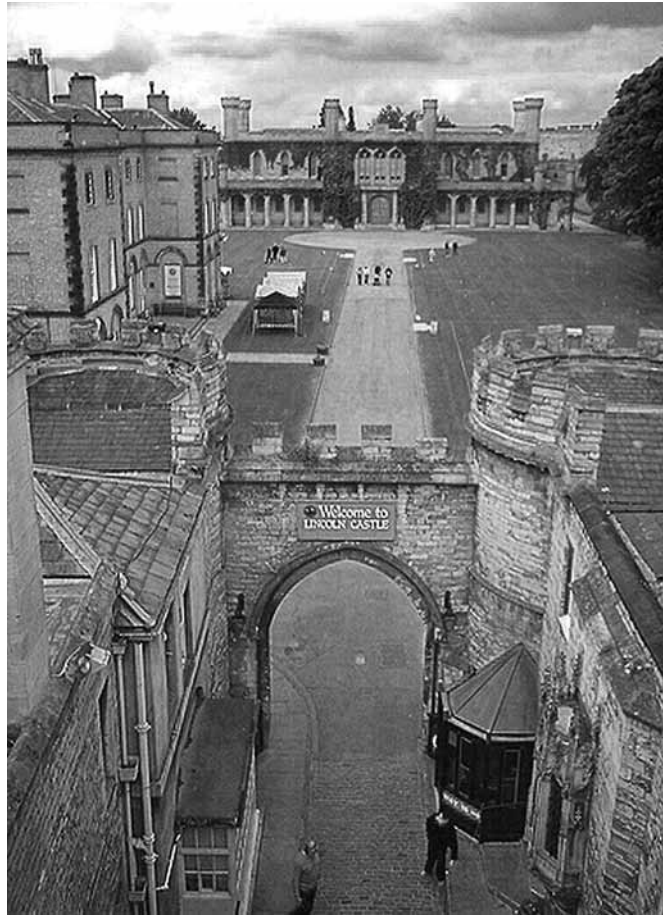
4.8 View of the Crown Court from above the east gate (photo by author)
