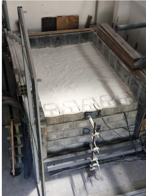
Fig. 1. View of a block-face wall at the end of construction.
