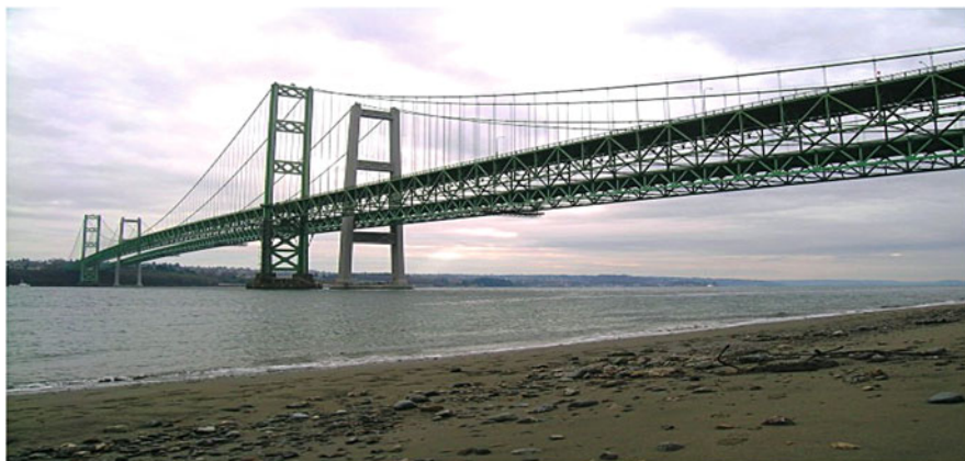
Fig. 1.13 The current twins Tacoma Bridges (1950 and 2007) (Reproduced with permission from Michael Goff, Oregon Department of Transportation, US, http://structurae.de/photos/index.cfm?id=100618 )
