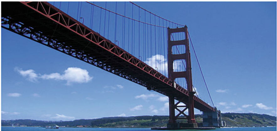
Fig. 1.12 The Golden Gate Bridge (1937) with its stiffening trusses (Source: http://commons.wikimedia.org/wiki/File:Golden_Gate_Bridge_from_underneath.jpg by Ambush Commander)
