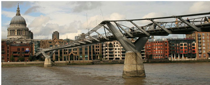
Fig. 1.6 The London Millennium Bridge (2000) (Reproduced with permission from Nadja Levtsenko, http://myself113.deviantart.com/art/Millennium-Bridge-97396006 )
