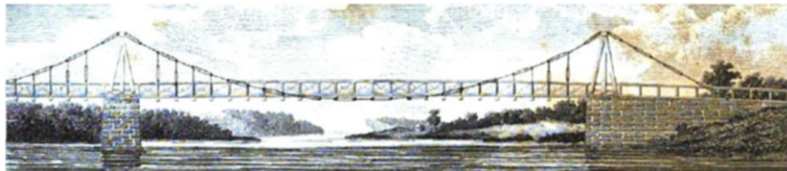
Fig. 1.4 View of the Jacob Creek Bridge (1801) (Source: [112, p.441], http://commons.wikimedia.org/wiki/File:Jacobs-creek-bridge-1.jpg )
