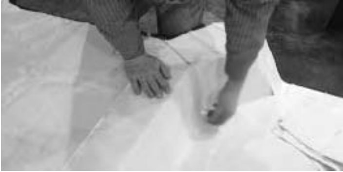
11.8 The angles are securely worked in to avoid bridging or bagging.
