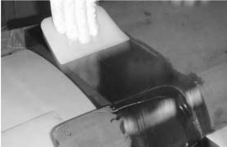
11.11 Spreading resin on carbon fiber.
