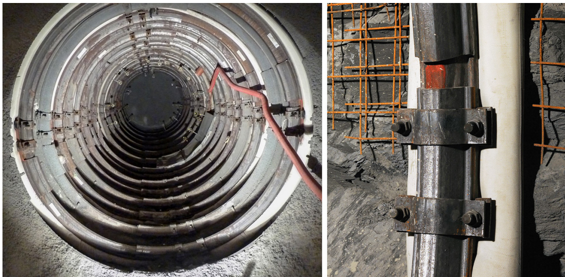
Fig. 4 The photo on the left shows the 12 m long shotcrete-free interjacent sealing section (ISS) at the end of the FE tunnel; the photo on the right shows a detail of a steel set bedded on a grout-injected hose for an even load distribution from the rock
