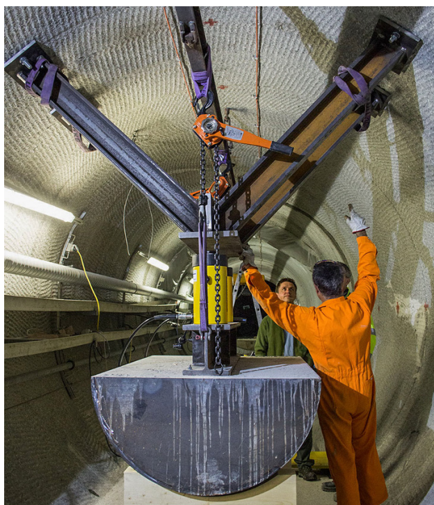
Fig. 12 Test set-up of the full-scale load test of a bentonite block pedestal at the Grimsel Test Site
