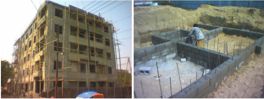
Fig. 4 In Chittagong, Reinforced Masonry (RM) proved to be even better and more economical than CM (pictures by the author)
