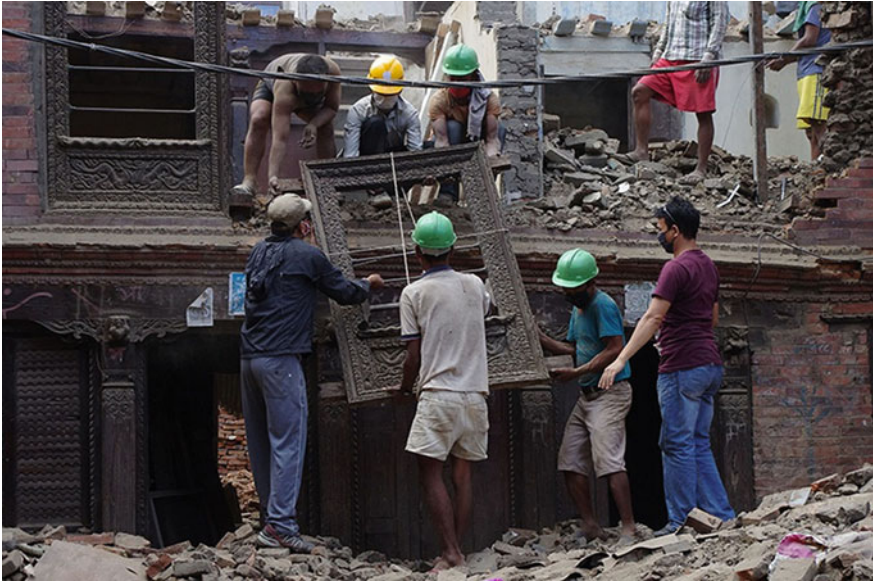
Fig. 2 Volunteers, students and workers taking extra care to remove the window frames
