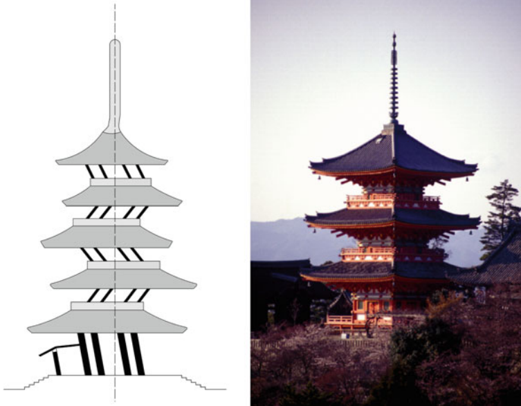
Fig. 10 Snake dance of the Japanese Pagoda during an earthquake. This rigid body motion balances the mass effects and thus limits the forces in the structure. The Pagoda System is the oldest (and highly proven!) seismic control system in the world (picture by the author)
