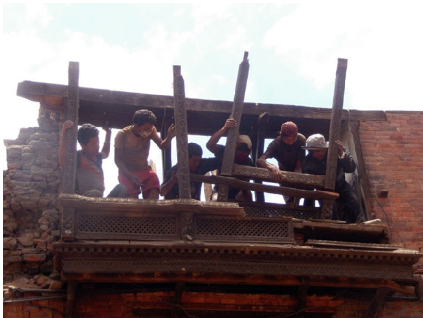
Fig. 4 Removal of the components of window with precision
