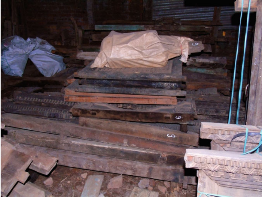
Fig. 6 Storage of wooden components of buildings with number coding for each building
