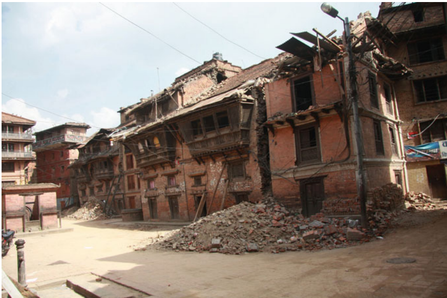
Fig. 1 Post earthquake situation in Gachhen, Bhaktapur
