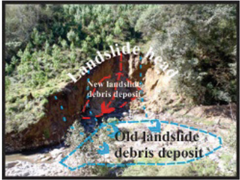
Fig. 6 Meader landslide. The blue line and arrows represent an old landslide debris deposit and landslide movement and the red line and arrow represent a new landslide debris deposit and movement
