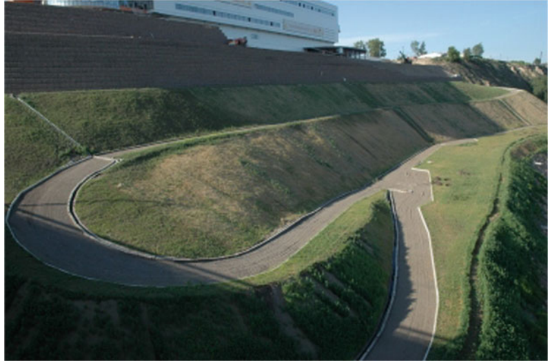
Fig. 21 After installation and commissioning of geohazards monitoring system
