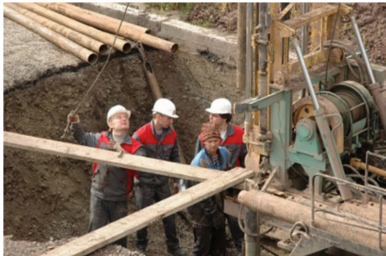
Fig. 17 Installation and commissioning of geohazards monitoring system
