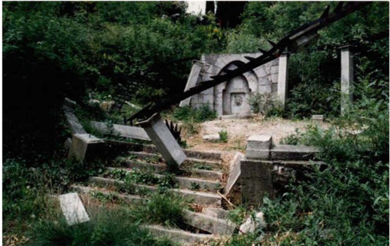
Fig. 8 The Laurel alcove destruction by the “West” landslide right border
