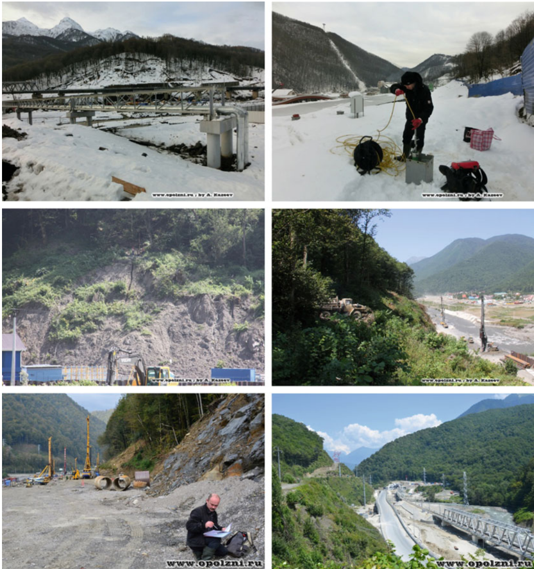
Fig. 15 The stages of works at railway Adler-Krasnaya Polyana construction
