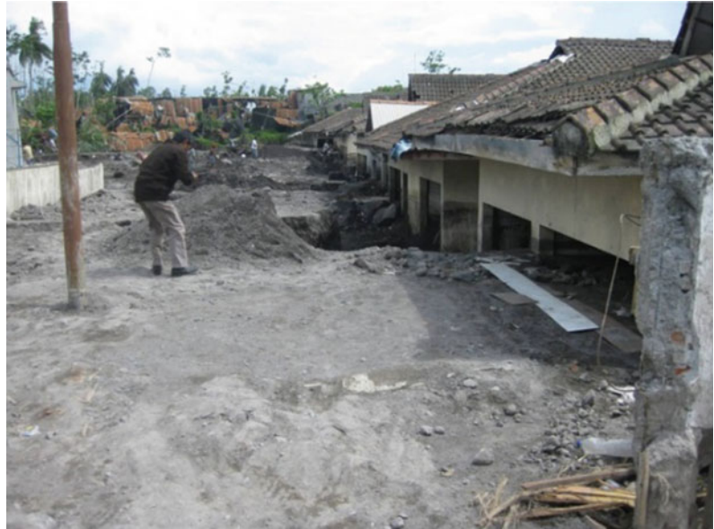
Fig. 3 Damage to houses near a river on the volcano
