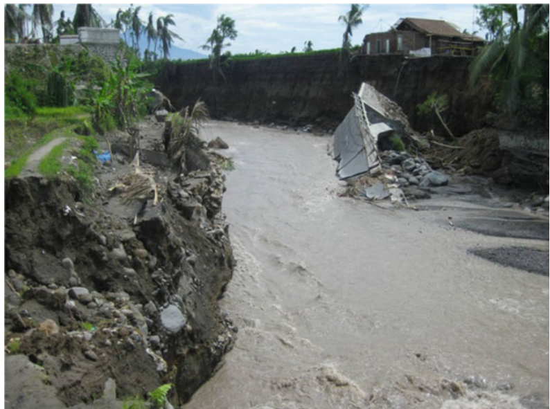
Fig. 2 Collapsed bridge due to the destructive power of a rainfall-induced debris flow
