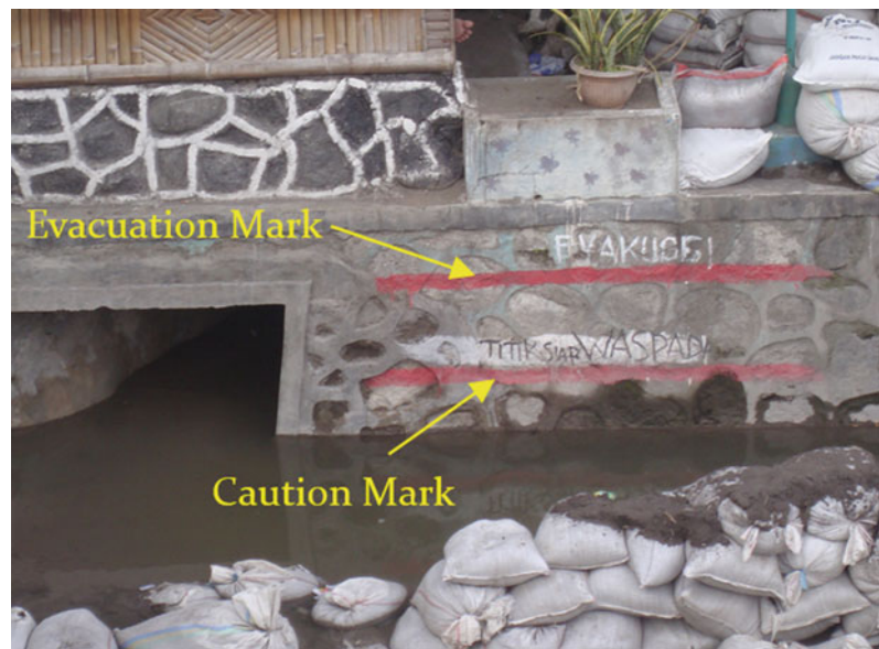
Fig. 9 Bank markings used for existing community warning alerts of debris flows
