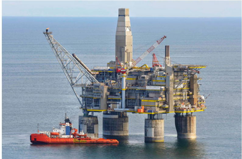
Fig. 9 Platform for PA-B deposit
