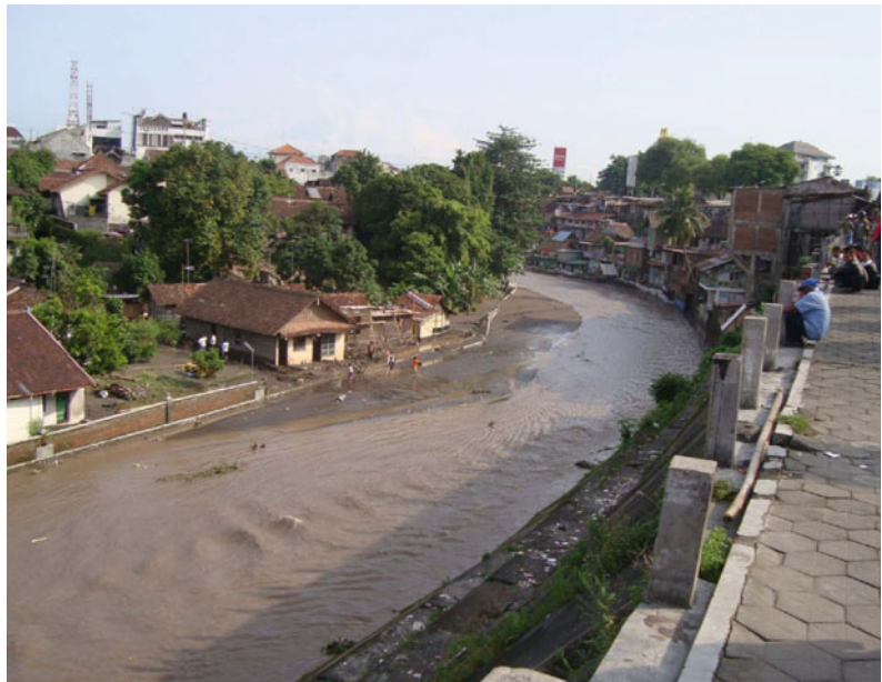
Fig. 6 Flow conditions of Code River downstream in the Jogoyudan area in Yogyakarta City on 30 November 2010
