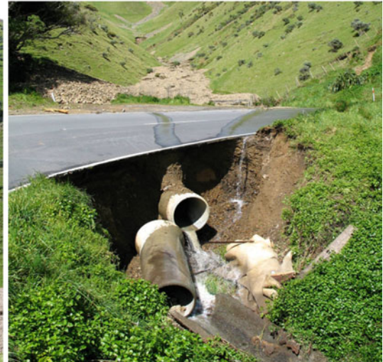
Fig. 3 Erosion gully and debris flood gravel deposits (a), and erosive effects of flood water on road-edge fill (b) at Paekakariki, October 2003 (from Hancox 2003)
