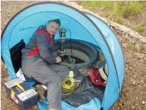
Fig. 19 Installation and commissioning of geohazards monitoring system
