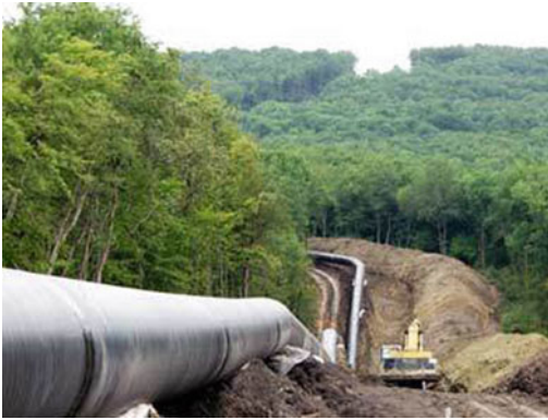
Fig. 5 “Blue Stream” during construction
