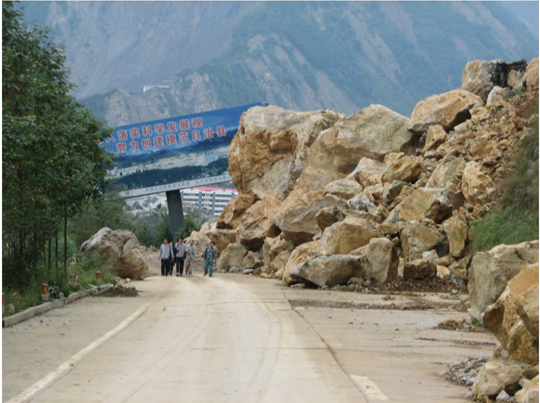
Fig. 6 A large rockfall due to the May, 2008 Wenchuan, China Earthquake. Rockfalls such as this one are often deadly, although rockfalls can involve small rocks, large
