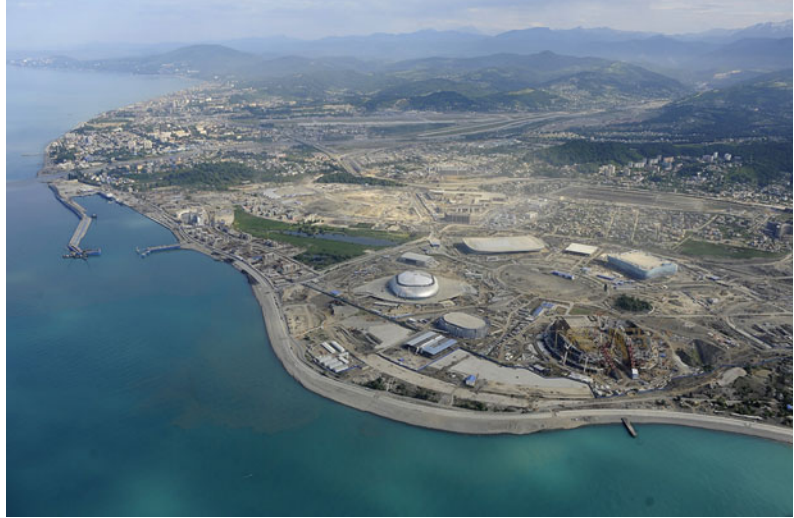
Fig. 9 Sea cluster. Imeretinskaya depression. Olympic objects during construction
