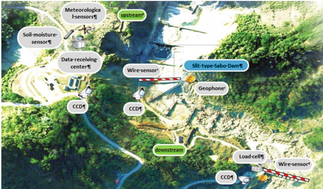
Fig. 16 Layout of sensors in Jioufen-Ershan monitoring station
