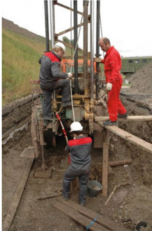
Fig. 18 Installation and commissioning of geohazards monitoring system
