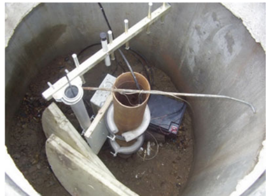
Fig. 20 Installation and commissioning of geohazards monitoring system
