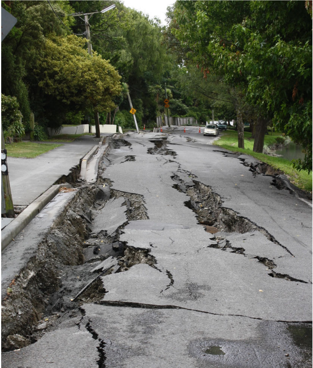
Fig. 19 The effects of lateral spreading in Christchurch, New Zealand as a result of the February 22, 2011 Christchurch Earthquake. Photo Wikipedia Commons.
