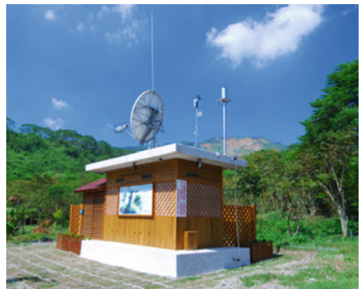
Fig. 12 Example of an on-site monitoring station
