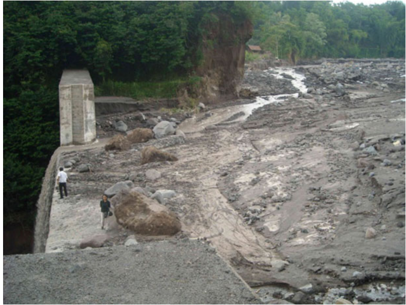
Fig. 5 Condition of the Boyong River upstream of Sabo dam BOD4 on 14 January 2011
