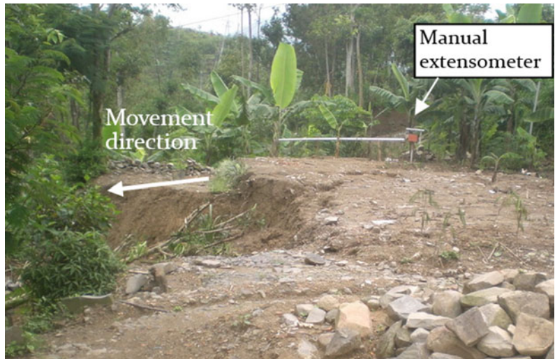
Fig. 4 Manual reading extensometer on the upper part of a collapsed slope
