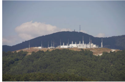
Fig. 7 The compressor station “Beregovaya”, view from the sea. Visible glade in which the buried pipeline
