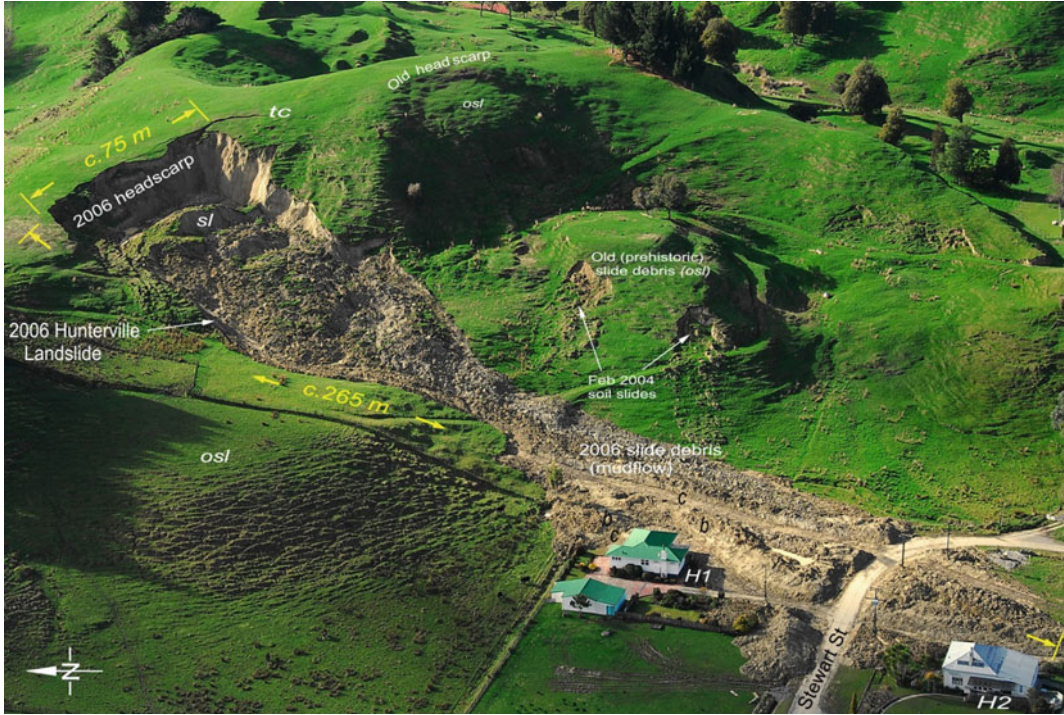
Fig. 7 Oblique aerial photo of the large (c. 5000 m 3 ), rotational slide ( sl ) and earthflow in mudstone, which threatened several houses ( H1 , H2 ) in Hunterville during a rainstorm in July 2006. The landslide, which formed on the headscarp of a ‘relict’ (prehistoric) landslide, is c. 75 m wide and 3–12 m deep at its head ( left ). It transformed into a slow-moving earthflow, which
