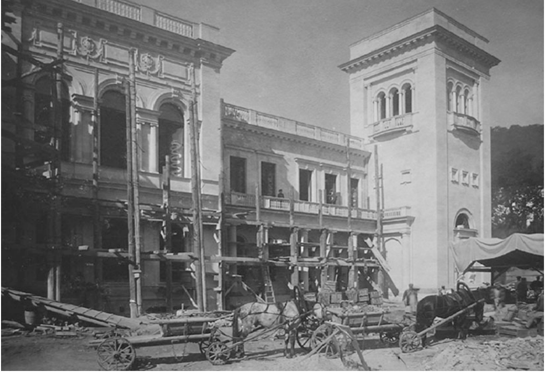
Fig. 3 The Livadia Palace construction
