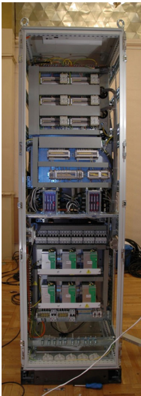
Fig. 6 UCP, view without back panel
