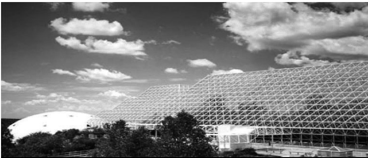
Figure 10.2 The dome of the project Biosphere II (picture edited from: http://upload.wikimedia.org/wikipedia/commons/d/d3/Biosphere2_1.jpg , accessed: 9 th July, 2014). The Biosphere II was an experiment conducted in the early 1990s. It was supposed to be a self-contained ecosystem with a team of scientists locked into it for 2 years. The 3.15 acre facility, made of glass and space-frame, was the largest total enclosed ecosystem ever built. All of the living things inside were taken directly from Biosphere I (i.e. the Earth). All seven ecosystems of Earth existed within the confines of Biosphere II. They were a rainforest, a desert, a savannah, a marsh, a farmland (in an area called the Intensive Agriculture Biome) and a 'human habitat'. Thus, it contained soil, air, water, animals and plants. About 4,000 plants and animals were introduced to Biosphere II and its ocean contained 3,400 cubic metres of water. It was hoped that these provisions would give the ecosystems enough material to be self-sustaining.
