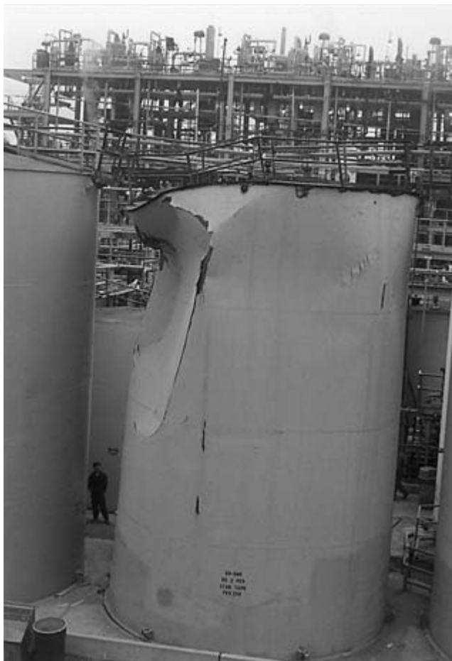
FIGURE 2-16 Crushed tank in the tank farm.
