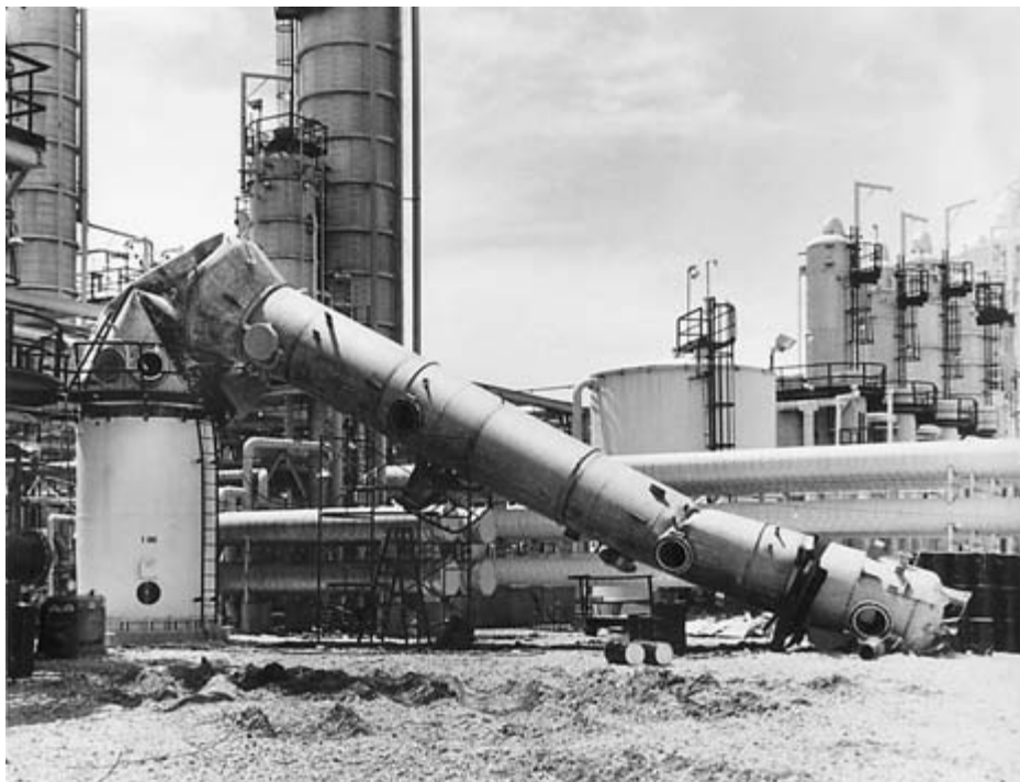
FIGURE 3-5 A stripper column collapses. Courtesy of Guido DeJesus.
