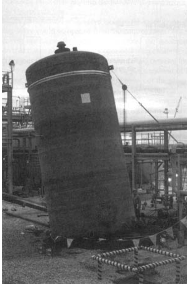
FIGURE 5-12 A large acid tank fails due to blocked vent and a blocked overflow line.
