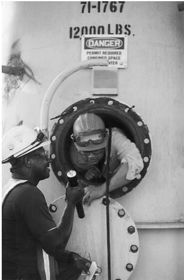
FIGURE 10–10 A pressure vessel inspector enters the confined space after the vessel is blinded, tested, and cleared, but still relies on a manway watch.
