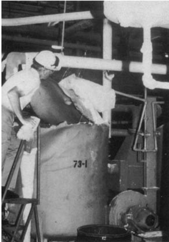
FIGURE 2-21 Employee examines the air dryer failure.
