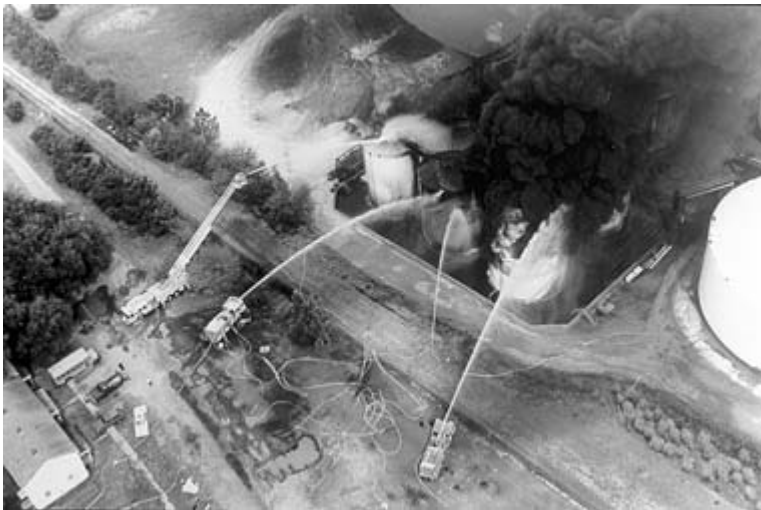
FIGURE 2-27 Fire Water Spray Cooling the Tanks. Courtesy of David Chung of the U.S. Environmental Protection Agency.
