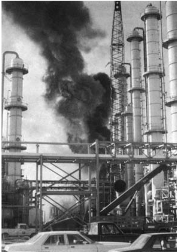
FIGURE 8-6 Fire in solvents plant as seen from the road. Courtesy of G. O. Heintzen.
