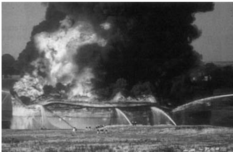
FIGURE 8-2 After the top opened, a fire burns and the liquid is still contained. Courtesy of the Institution of Chemical Engineers. This photo is available in IChem's Hazard Workshop Module No. 3, "Fires and Explosions."
