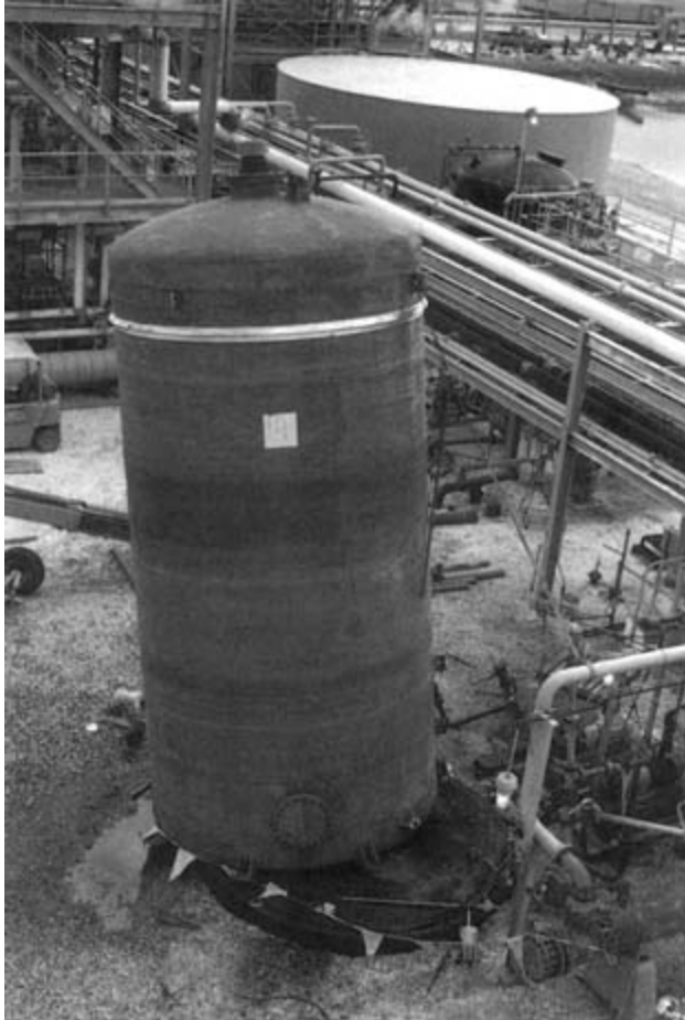
FIGURE 5-13 An aerial view of the tank failure.
