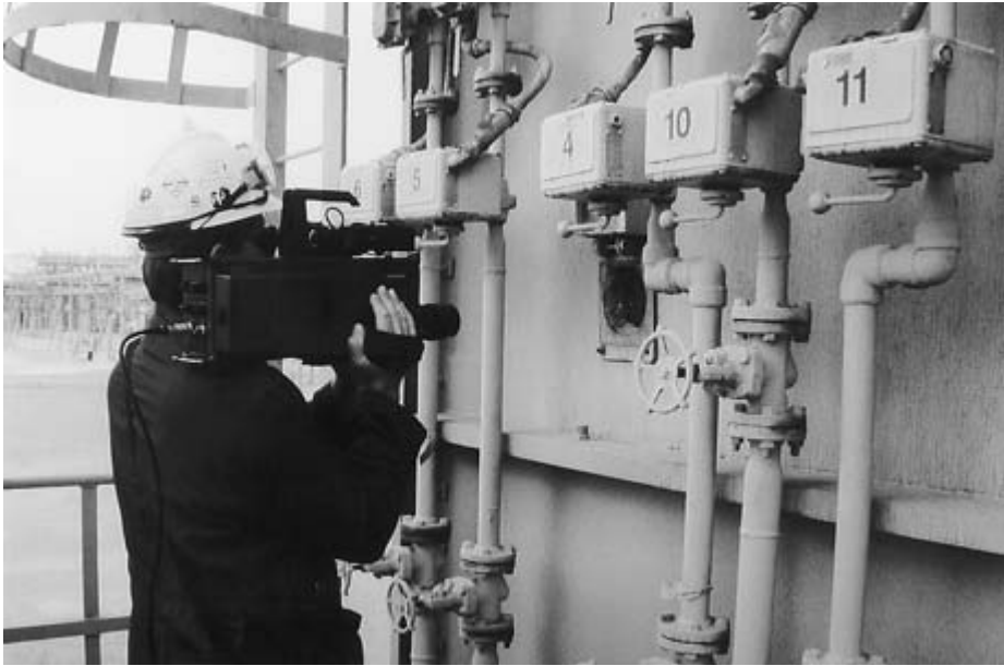
FIGURE 10-5 An inspector using an infrared camera periodically monitors furnace tube temperatures through the inspection port holes.
