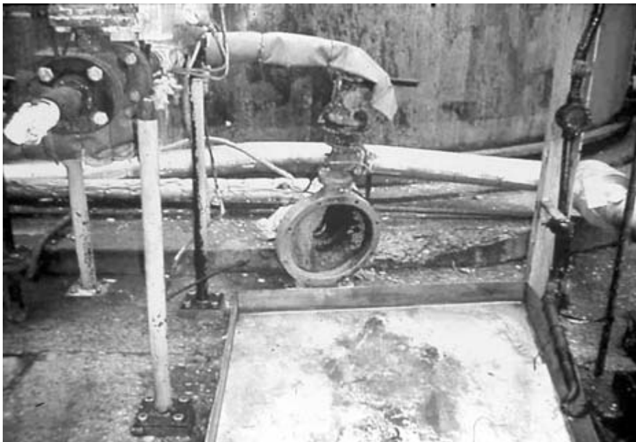
FIGURE 7-12 Pump bowl is stripped of the pump and base plate. Courtesy of Eastman Chemical Company.
