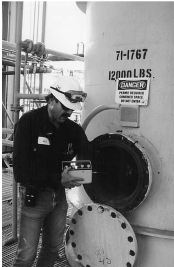
FIGURE 10-8 An operations foreman checks for blinding and samples the vessel's atmosphere before tank entry.
