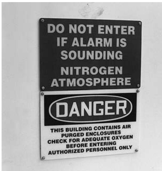
FIGURE 2–24 Signs found on the typical pressurized and purged analyzer buildings found in chemical plants handling flammables.
