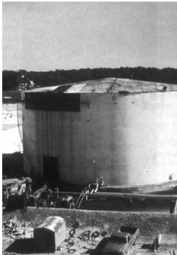
FIGURE 6-12 Repairs in progress on a large tank.
