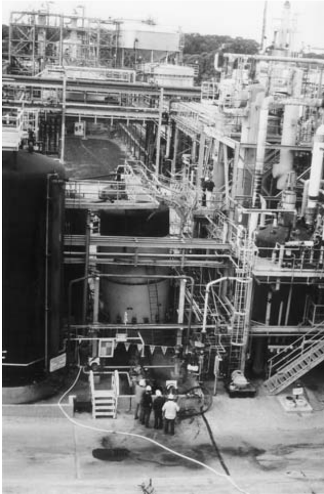
FIGURE 3-1 An API 620 tank is damaged during a hydrotest.
