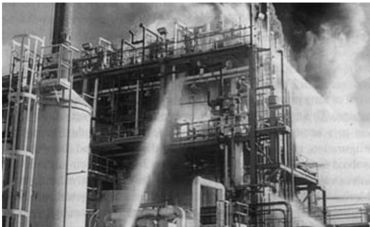
FIGURE 8-7 Fire intensely burning in the reactor area in the third level of structure, while hose streams supplement the fixed water spray. Courtesy of G. O. Heintzen.
