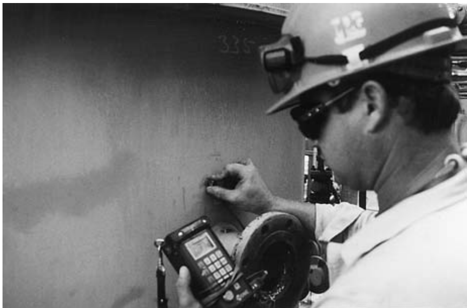
FIGURE 10–11 An inspector verifying wall thickness on a vessel near a nozzle that had experienced metal loss.
