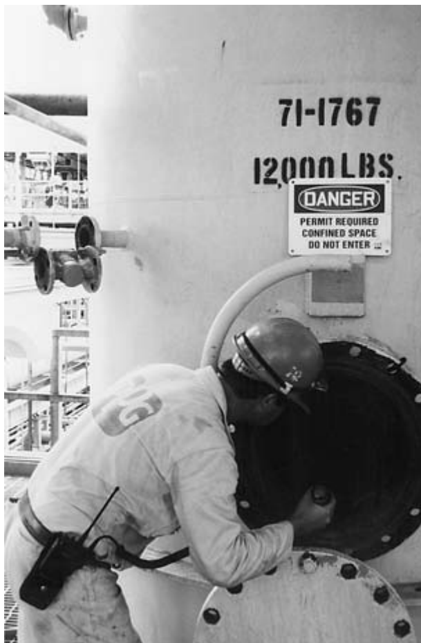
FIGURE 10-9 A pressure vessel inspector making an initial assessment of the vessel and determines any special inspection needs, such as ladders, scaffolding, or extra lighting.
