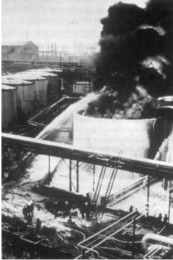
FIGURE 8-3 A fire in a giant floating roof crude oil tank. Courtesy of the Institution of Chemical Engineers. This photo can be found in Hazard Workshop Module No. 6, "Preventing Emergencies in the Process Industries, Volume 1."
