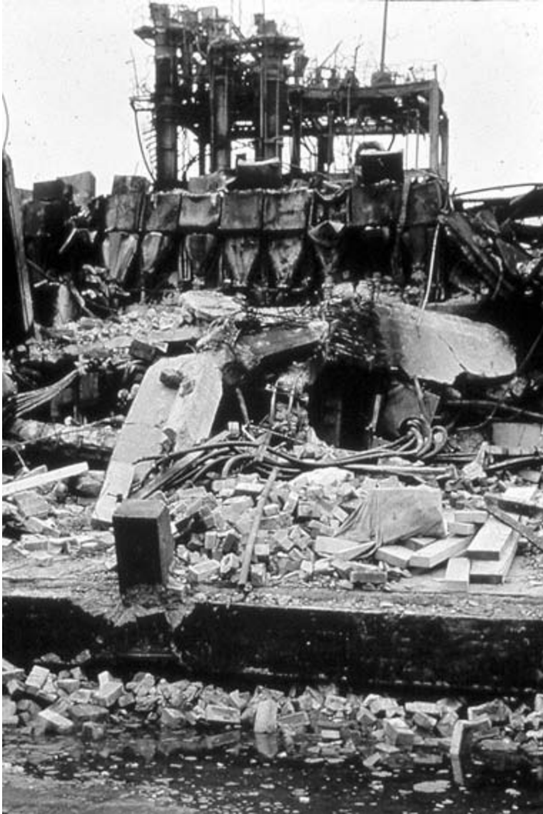
FIGURE 5-17 The rubble of the crushed control room at Flixborough. Courtesy of Trevor A. Kletz.
