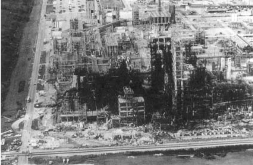
FIGURE 5-5 Aerial view of the charred structure and destruction at Phillips 66. Courtesy of Factory Mutual Research Corp.
