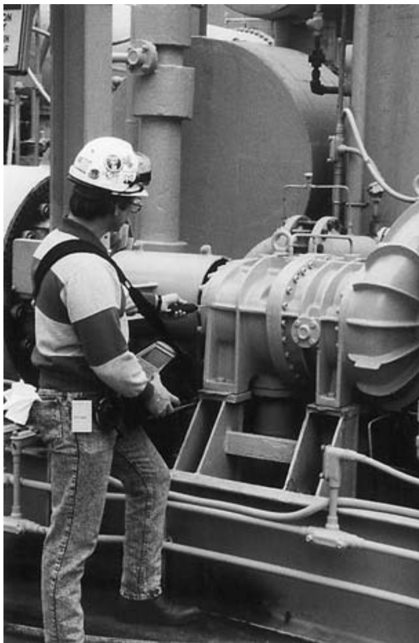
FIGURE 10-3 A vibration technician taking readings on a refrigeration compressor.
