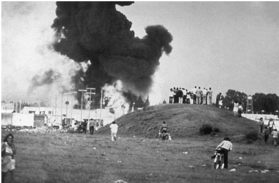
FIGURE 5-10 BLEVE of a vinyl chloride storage tank. Courtesy of the Institution of Chemical Engineers.
