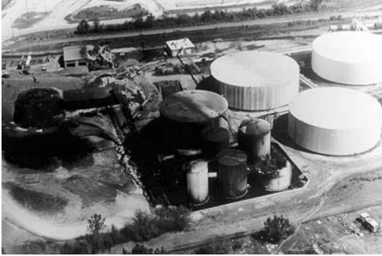
FIGURE 2-28 Burnt Out Tanks and Terminal. Courtesy of the U.S. EPA.
