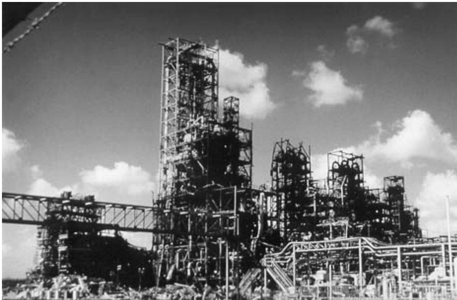
FIGURE 5-6 A ground-level view of the charred structure and destruction at Phillips 66. Courtesy of Factory Mutual Research Corp.
