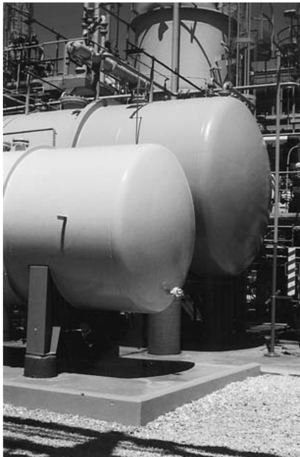
FIGURE 10–7 Well-maintained pressure vessels (over 30 years old) still safely handling hazardous materials.
