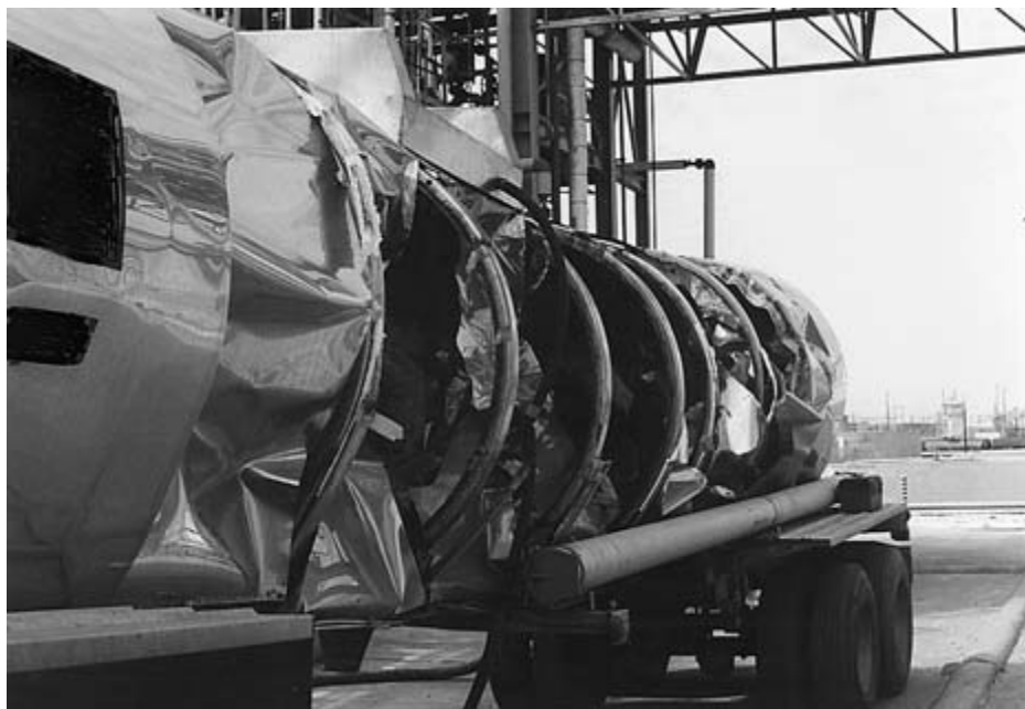
FIGURE 2-5 Close-up of tank failure and exposed ribs.
