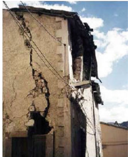
Fig. 20.37 Combined overturning of a multi story wall (Milano et al. 2008)
