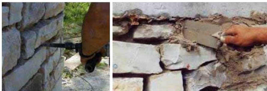
Fig. 20.70 Execution phases of the repointing intervention
