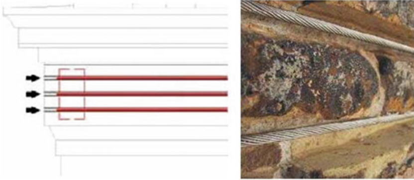
Fig. 20.53 Example of steel strand hoops
