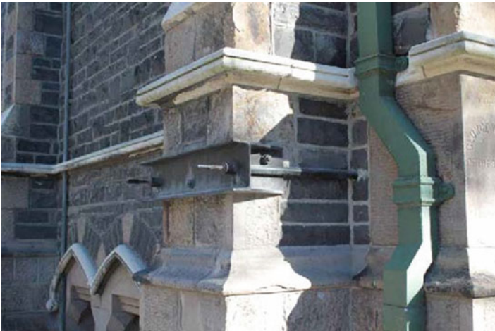
Fig. 20.54 Horizontal post tensioned ties in a masonry building in Christchurch that withstood the 2011 earthquake
