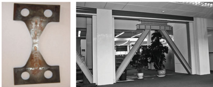
Fig. 17.5 Example of ADAS dampers
