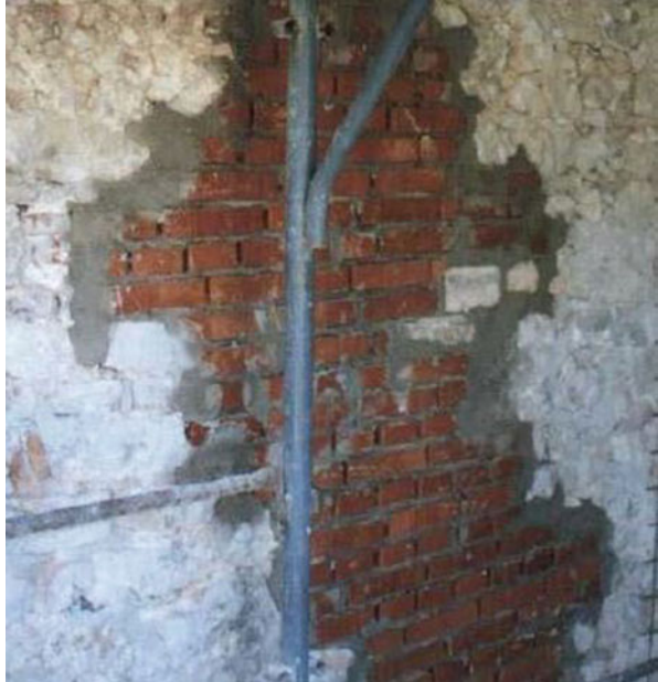
Fig. 20.62 Example of patching
