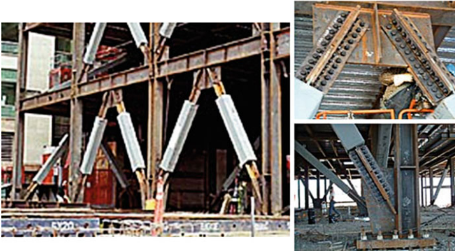
Fig. 17.15 Example of BRB dampers implementation
