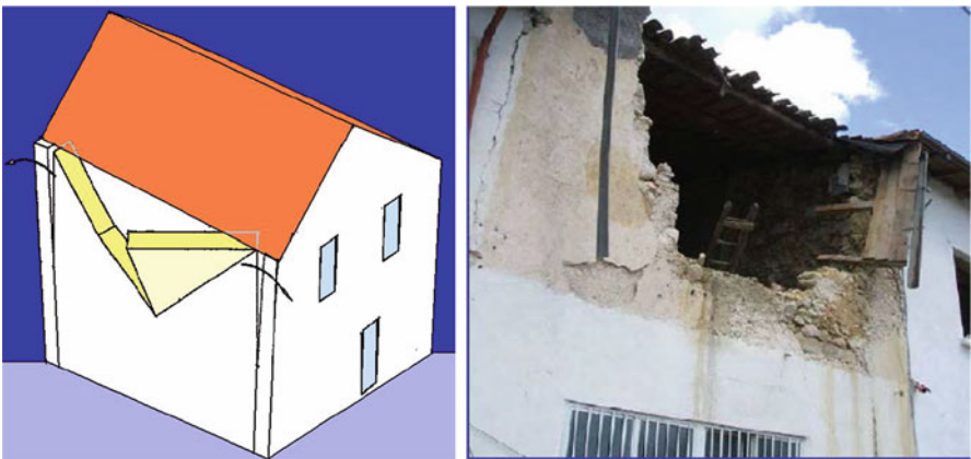
Fig. 20.40 Horizontal flexure (Milano et al. 2008)
