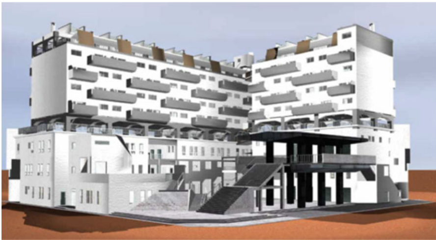
Fig. 19.29 Building located near Tokyo
