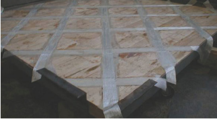
Fig. 20.60 Application of FRP stripes at the extrados
