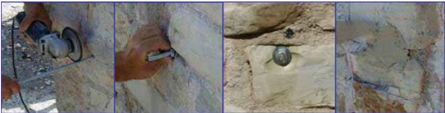
Fig. 20.63 Phases of laying the connectors
