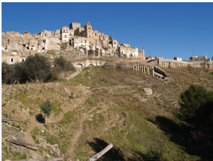
Fig. 5.1 Recent composite landslide occurred in 1972 on the southern versant of the hill of Craco, Province of Matera, Southern Apennine, Italy. The town, of medieval origin, was located upon an arenaceous block overlying grey clays of Medium-Upper Pliocene
