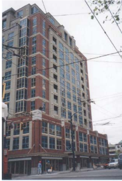
Figure B.1 North building face from Robson street
