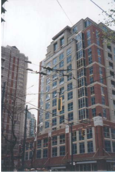
Figure B.2 East building face from Hamilton street
