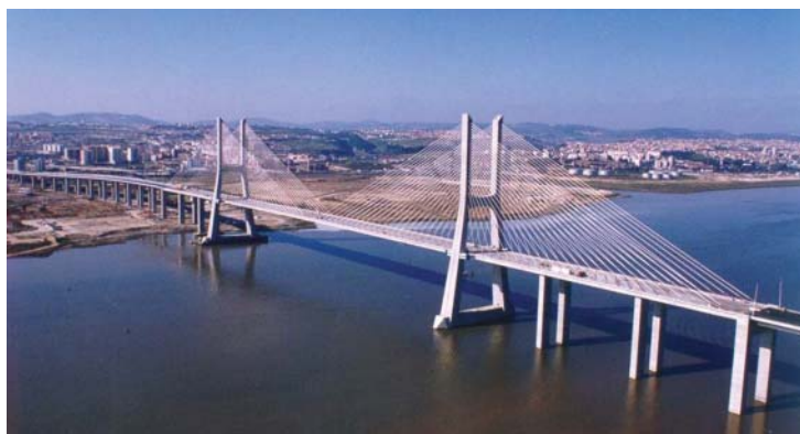
Figure 11.11 Overall view of the Vasco da Gama cable-stayed bridge (Source: Courtesy of Cuhna, et al. [13])
