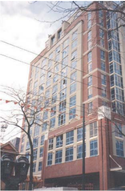
Figure B.3 South building face from Hamilton street
