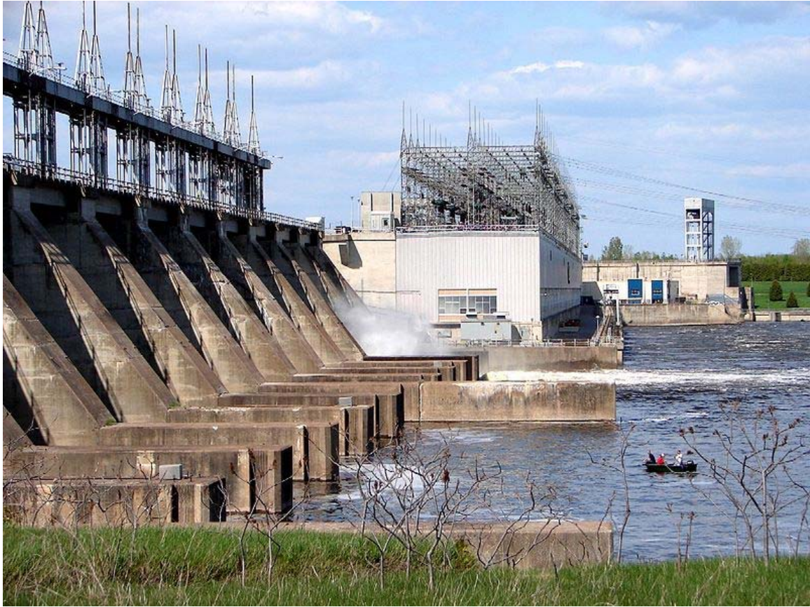
Carillon power station and dam
