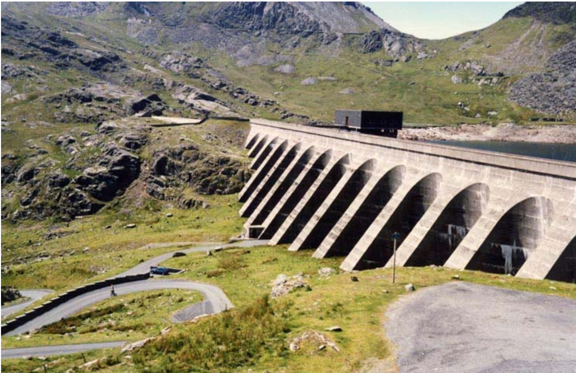
The upper reservoir (Llyn Stwlan) and dam of the Ffestiniog Pumped Storage Scheme in north Wales. The lower power station has four water turbines which generate 360 MW of
