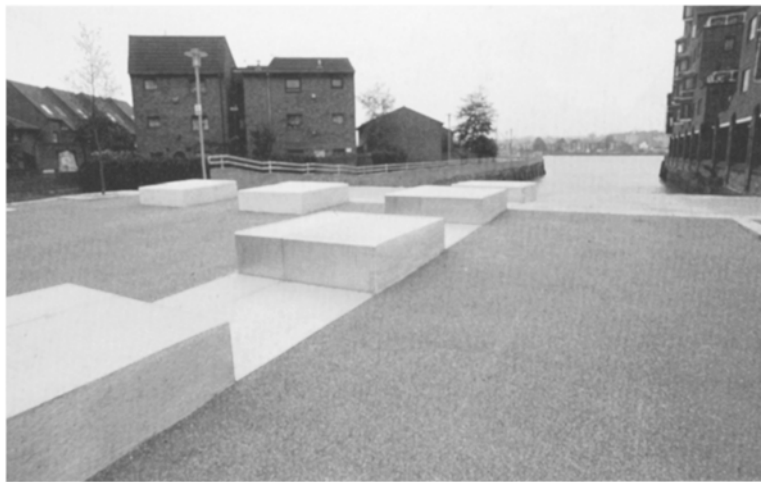
12 Plinths rising up to and marking the flood defence threshold. (Photograph © Martin Jones Photography)
