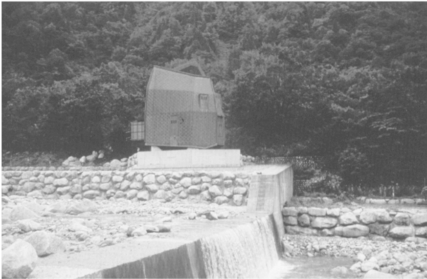
5 North elevation of the Kamiichi Mountain Pavilion sitting on a plinth above the flood level at the edge of a melt water river.
