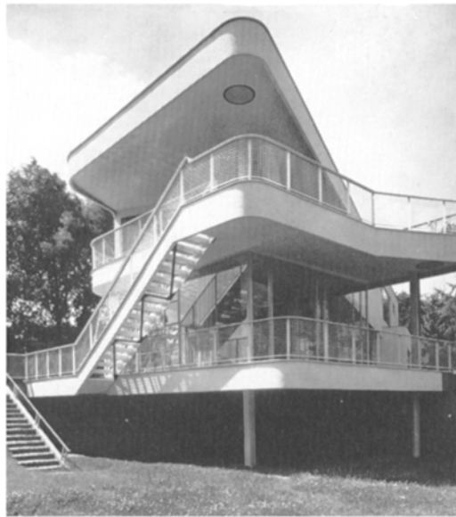
4 House from North, showing projection over garden. (Scharoun Archive, Akademie der Künste)
