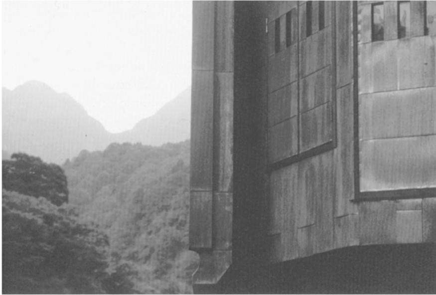
6 Detail of the copper shell of the Kamiichi Mountain Pavilion, showing Bambajina beyond. (Photograph Peter Salter)
