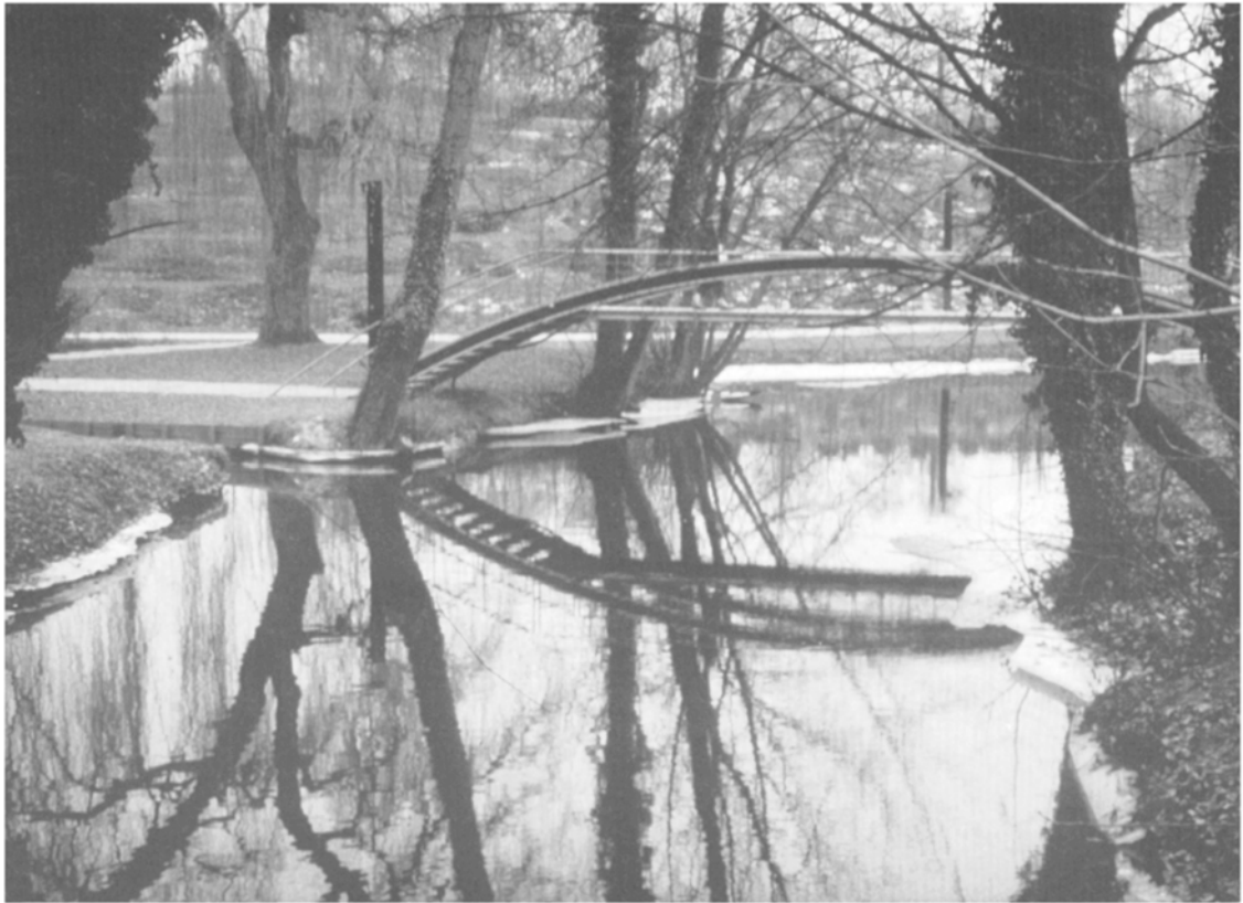
6 Bridge over the Bras Baraban connecting the northern and southern parts of the park. (Photograph Sandra Morris)
