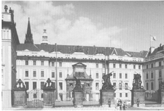
3 First Castle Court, Prague Castle: Matthias Gate (1614); facades by Niccolo Pacassi (1763–1761); flagstuffs and paving by Jož Plenik (1922–1923). (Photograph Caroline Constant)
