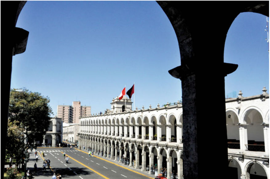
Fig. 6.13 Impressive historical buildings in the main square of Arequipa built with white volcanic rock blocks Credit Menegat and Fontana
