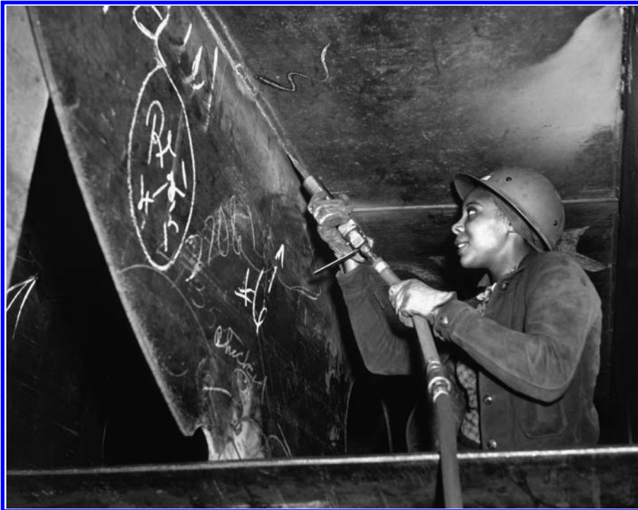
FIGURE 1.12 Scaler Eastine Cowner, Liberty Ship construction. (From http://www.dodmedia.osd.mil/DVIC_View/Still_Details.cfm?SDAN=HDSN9902466&JPGPath=/Assets/Still/1999/DoD/HD-SN-99-02466.JPG . Author: E. F. Joseph, US Office of War Information. Source: WikiCommons.)
