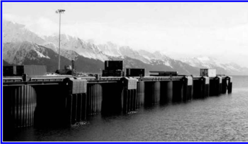
FIGURE 9.A10 Open Cell bulkhead dock with fenders. (Courtesy of John W. Pickering, PE, MBA, President, PND Engineers, Inc.)
