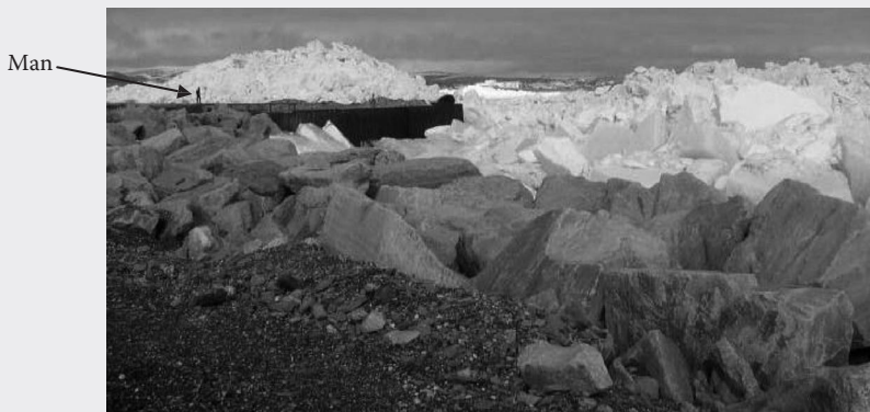
FIGURE 9.A11 Man standing on Open Cell dock overtopped with wind-driven sea ice, Nome, Alaska. (Courtesy of John W. Pickering, PE, MBA, President, PND Engineers, Inc.)
