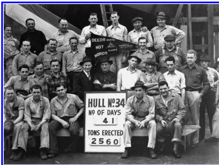
FIGURE 1.10 “Deeds, Not Words”. Twenty-eight male Delta Shipyard company workers in New Orleans, Louisiana during WWII, building Liberty Ship’s Hull Number 34 of 2,560 tons in 41 days. (Courtesy of the National World War II Museum, New Orleans. Images Gift of Earl and Elaine Buras, 1999. )
