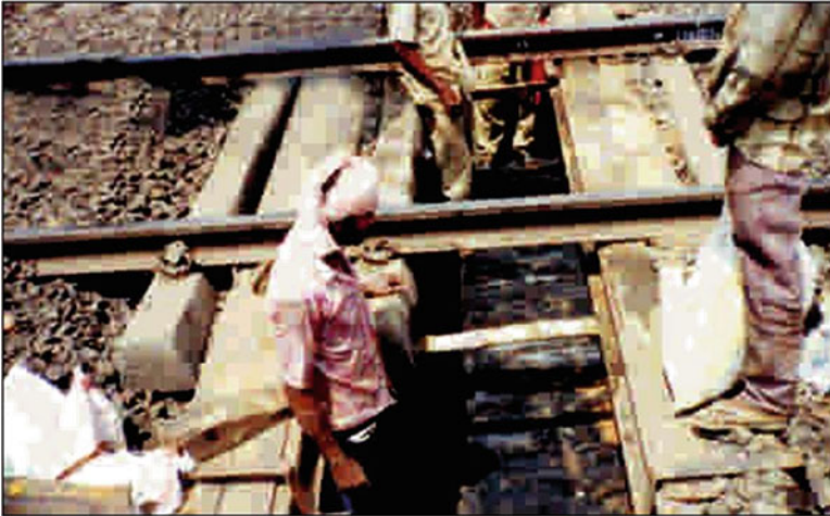
Fig. 17.14 Laying of JGT (woven and nonwoven)
