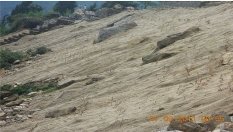
Fig. 17.22 JGT installed over slope
