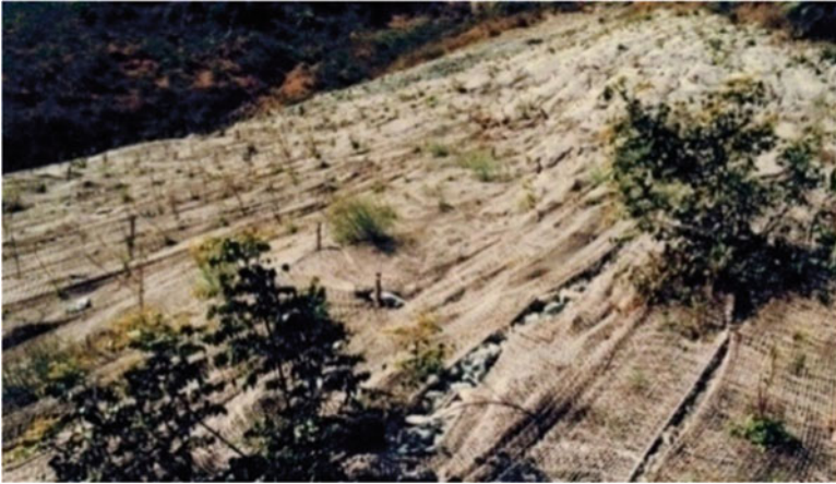
Fig. 17.19 JGT laid over the heap
