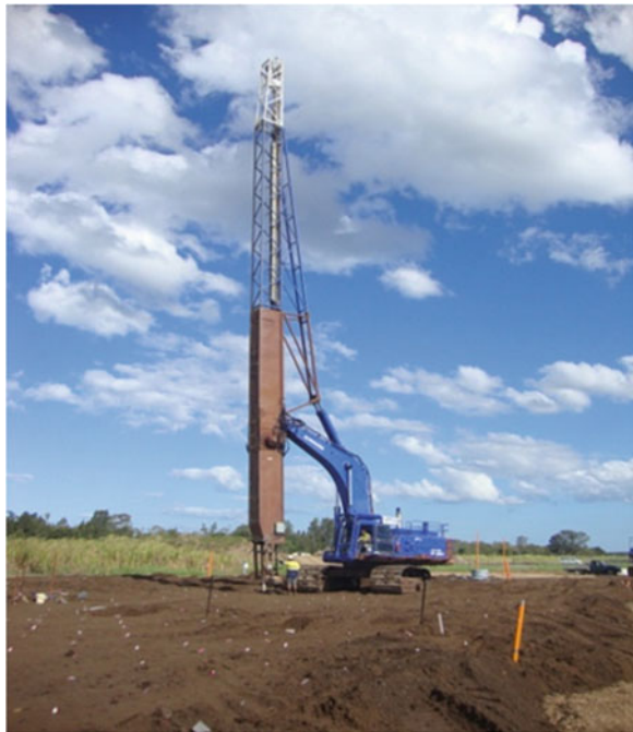
Fig. 10.2 Installation of PVJD in progress in Ballina, Australia
