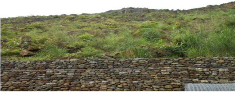
Fig. 17.24 Stabilized slope after reclamation with JGT
