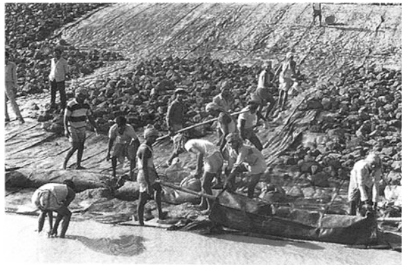
Fig. 17.9 Riprap laying in progress
