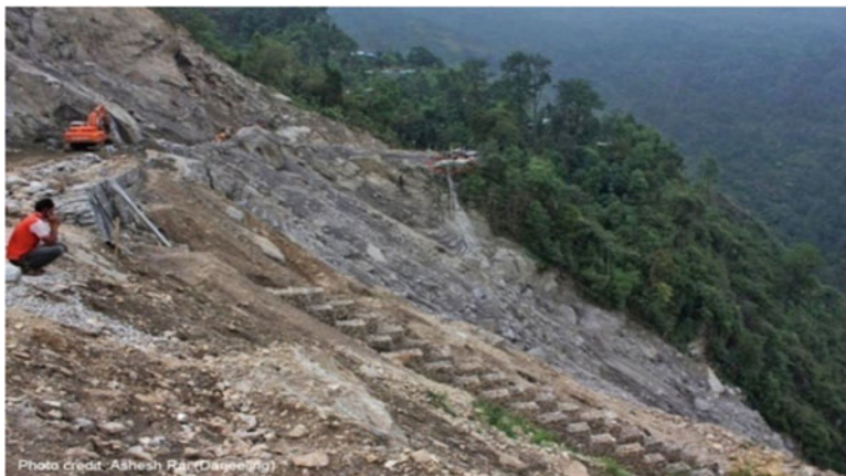
Fig. 17.23 Cascading in progress
