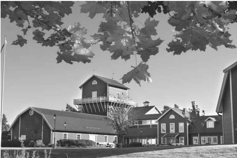
Figure 16.1 Surface buildings of the SKB Åspo Underground Rock Laboratory for radioactive waste management research near Oskarshamn, Sweden (Source: SKB)
