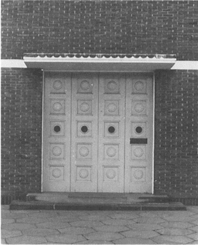
Holfordian detail from the central administration buildings at Team Valley.
