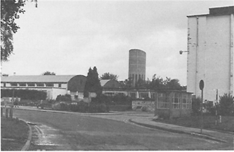
British Telecom Training College, Stone. The concrete water tower is a later addition.
